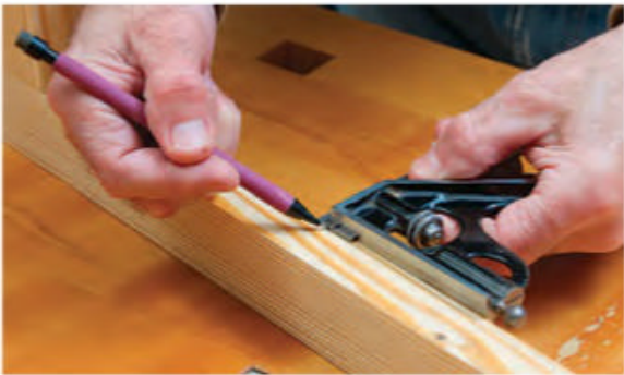
The inward facing lattice grid (the side that faces into the room) is permanently attached to the frame. Establish the grid's 1/8" setback with a combination square and pencil.
