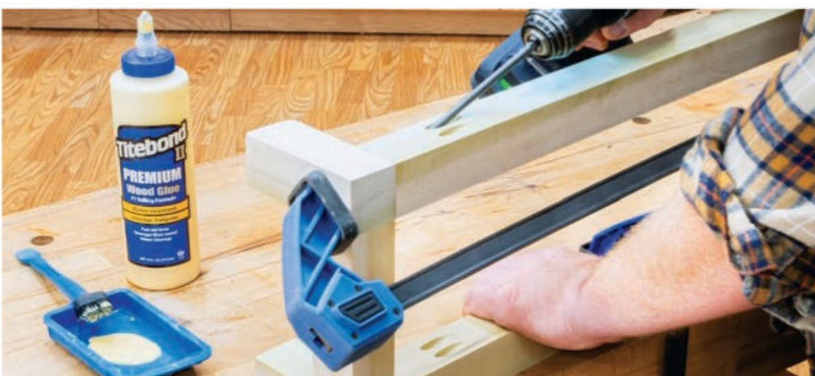
Poplar is a sturdy paint-grade hardwood for this bookcase's base. Assemble the legs and stretchers with glue and pairs of pocket screws at each joint. Orient the screw pockets to hide them.
