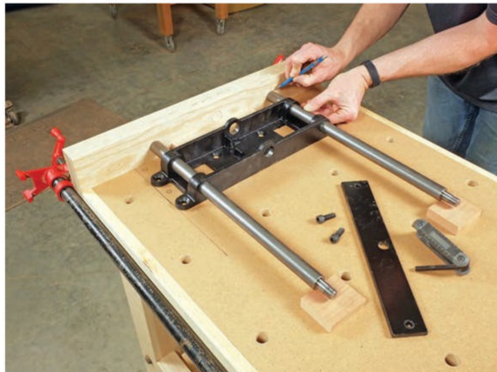
To install the tail (or side vise), first clamp a wooden vise face into place and set the vise's base into position. Reverse the guide rods in the base, and trace their locations and the center screw position onto the vise face.
