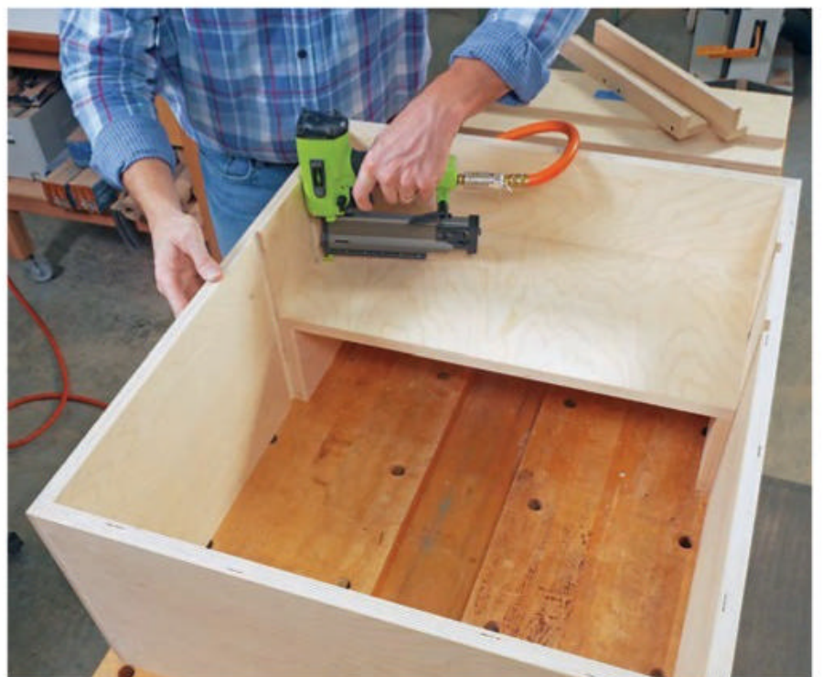
Glue and brad-nail the lower blocking pieces to the lower inside back corners of the cabinet. Then sand the front face of the lower back panel, fit it into place and nail it to the front edges of the blocking.
