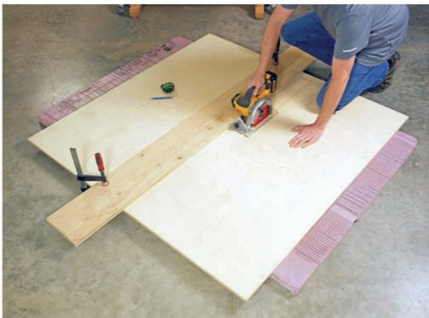
Splitting large sheets of heavy 3/4" plywood down into smaller, more manageable pieces is often safer and easier to do with a circular saw and clamped straightedge rather than a small jobsite table saw.
