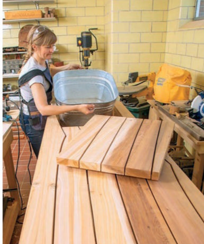
The client’s galvanized bin fits down inside the bench and wedges against a pair of inner cross braces. A slatted lid, shown here, covers the bin opening in the top.
