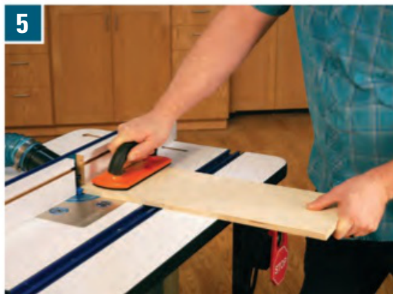
5 Rout the drawer lock profile across both ends of the back panel — the face against the router table will become the inside back face of each drawer. We made these cuts into a double-wide blank of 1/2" plywood to improve stability during routing and to help speed up the process. Once the joints are cut, you can rip the panel to form both drawer backs.
