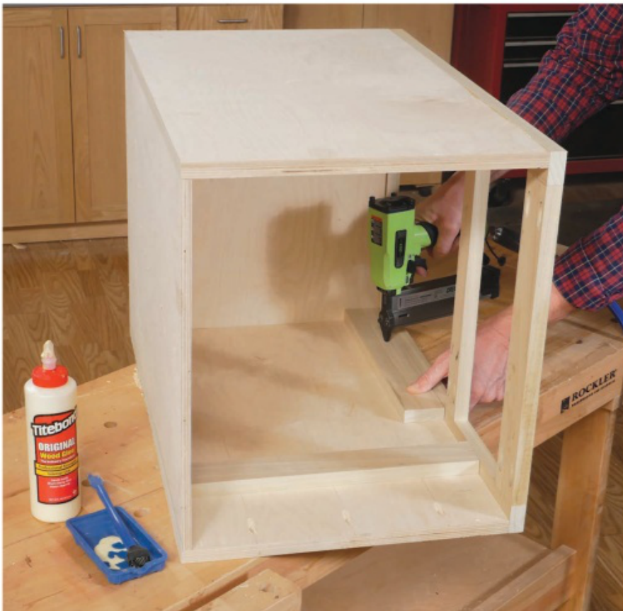
A pair of slide supports and a hinge mounting plate (being fastened in place here with glue and brad nails) raise the drawer slides and door hinge hardware so they're flush with the face frame openings.
