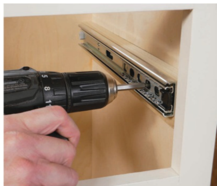
Full-extension drawer slides like these have numerous slotted screw holes so they can be installed and then adjusted as needed.
