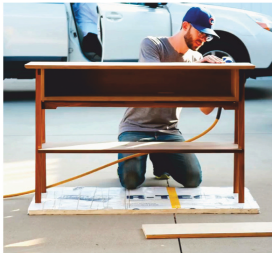
While the glue was curing on the drawer assembly, the author moved on to attaching the back panel with pin nails.
