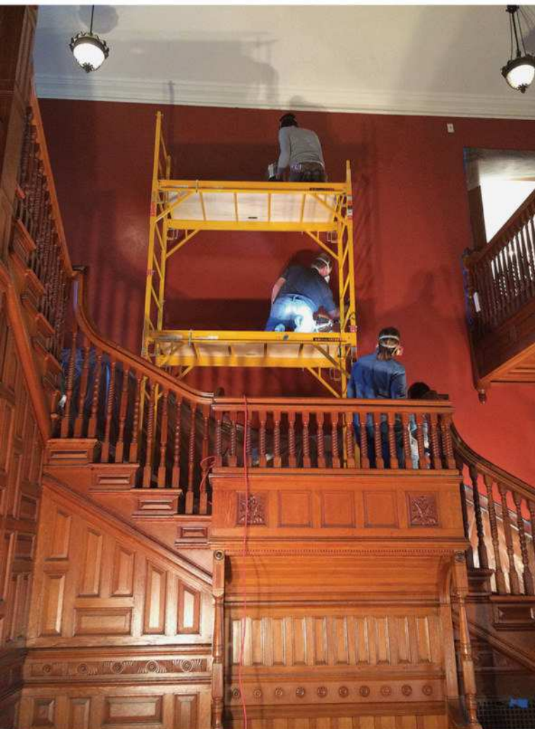
The main hall staircase extends for three stories. Paint restoration throughout the house required techniques such as hand grinding pigments.
