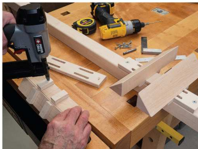
Use the slotted platforms to establish the space between the brace guides, and then fasten the guides to the bottom of the rear wheel braces. The author used a pin nailer (optional) and glue.
