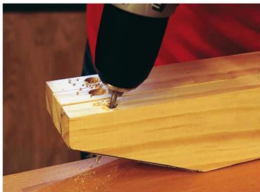
Drill pilot holes at an angle through the tops of each of the legs. Start with a 3/8" bit to create a counterbore, then finish the pilot hole with a smaller bit.
