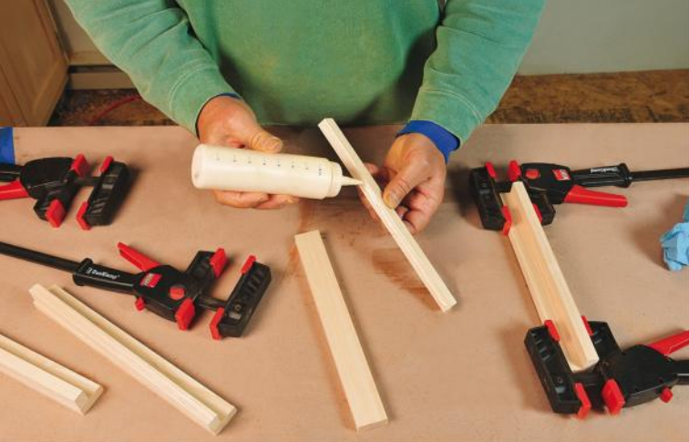
Glue up the picnic basket's four frame stiles using two pieces of stock to form a corner that's "L" shaped in cross-section. After the frame is assembled, round these corners over.
