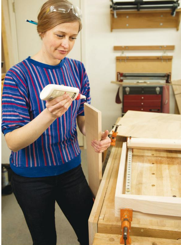
Glue and clamp together the cart's two trays, then the tray support assembly, before gluing up the rest of the cart.
