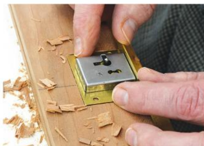
Check the depth of the initial mortise by setting the lock in place upside down.
