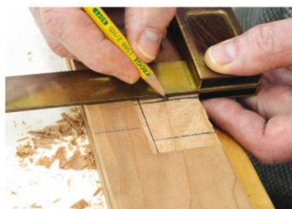
Measure and mark the initial mortise for the secondary mortise that will accept the body of the lock.
