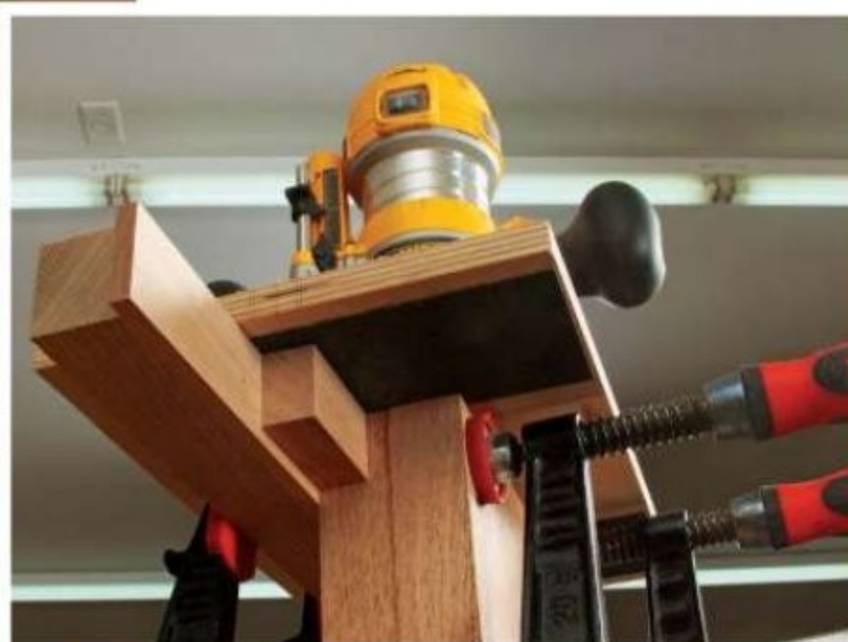
Routing mortises into the ends of the long bed rails required clamping them on-end in a bench vise. Double them up to provide better support for the mortising jig. Adding a 1/4"-thick shim and stop block (inset) enabled the same leg mortising jig to produce the rail mortises, too.
