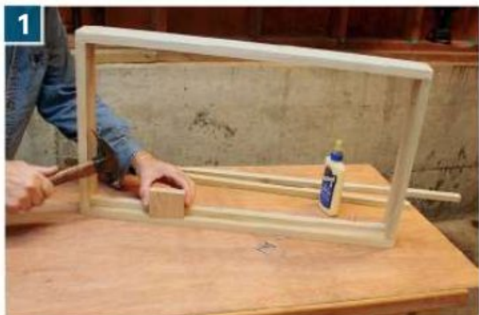
1 Install ledges inside the table framework to support the bottom plywood layer. Use a scrap depth gauge to locate the ledges accurately.
