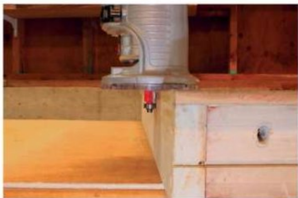
Trim the laminate and MDF layers even with the outside edges of the router table frame using a piloted flush-trim bit.
