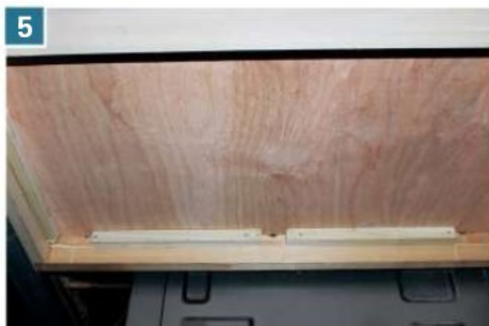
5 Notice that initially, the plywood layer will block access to the bolt holes when resting on the ledges.
