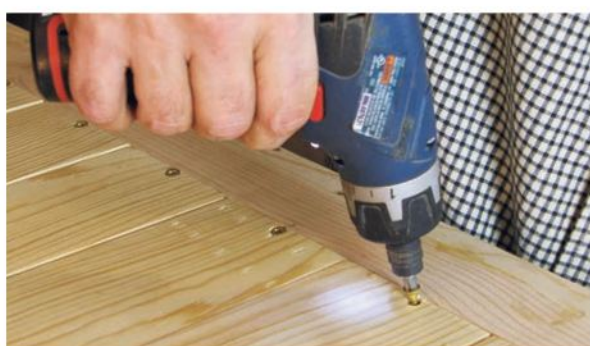
The back slats were secured to the carcass by a single screw at each end of the slats. The author chose to gang-cut the notches into the shelf stiles on his band saw (below). The primary advantage to that technique was to save time both on marking out the shelf stiles and in cutting all the notches.
