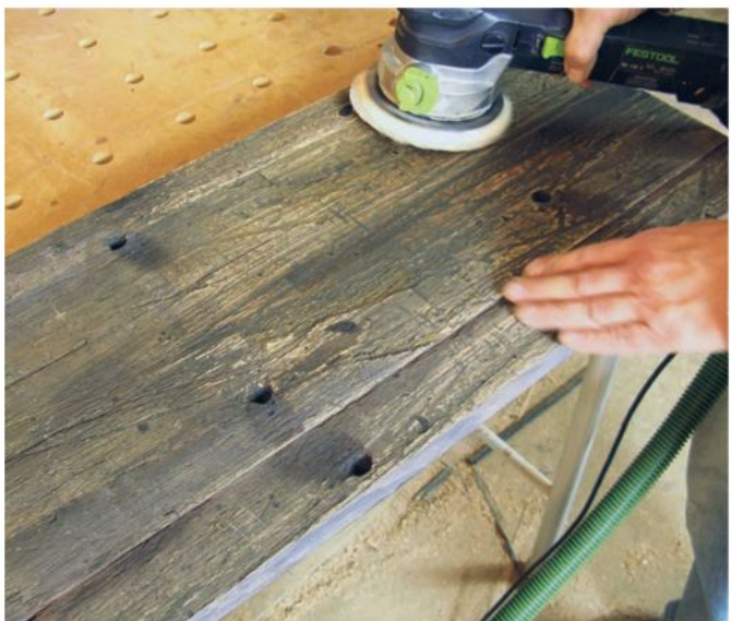
A light sanding with 100-grit paper on a rotary sander brought out highlights of the oak hidden by the ultra-dark patina (above). Soaking steel wool in white vinegar creates a solution that will darken oak by reacting with tannin in the wood fibers. The results on these pieces matched the exposed oak edges to the recycled lumber.
