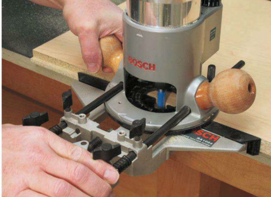
Photo 1: Get started by routing the 1/4" x 1/2"-deep rabbets in the sides (pieces 3) to accept the back (piece 5). Use a 1/2"-diameter straight bit and edge guide.
