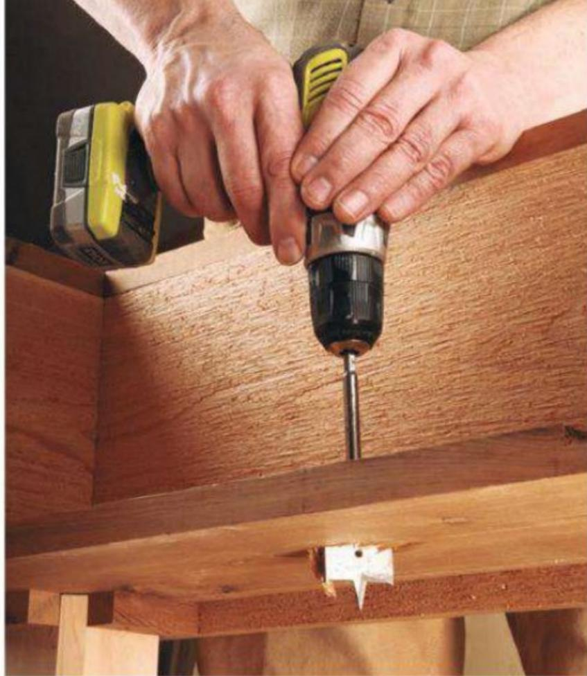
**Because the plants will need to be watered, bore drainage holes in the cross braces. The author used a 1/2" paddle bit to make the openings (upper left). Below, brad nails secure the decorative trim.**
