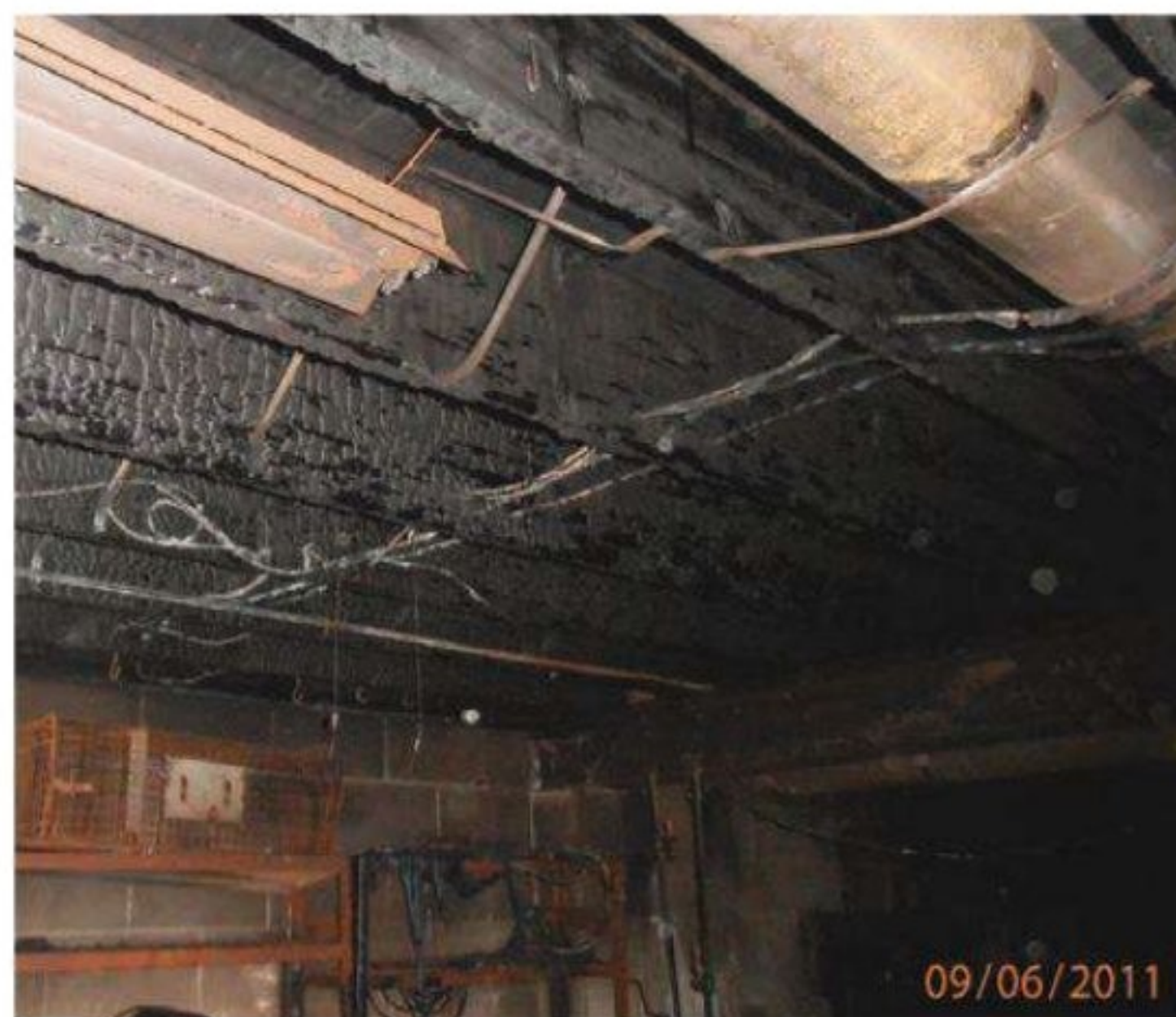
Woodworker Mark Thiergartner lost his house when a fire started in his basement. Wood and other fuel products caught fire in very short order. Burned joist, clamps and a router are just part of his loss.
