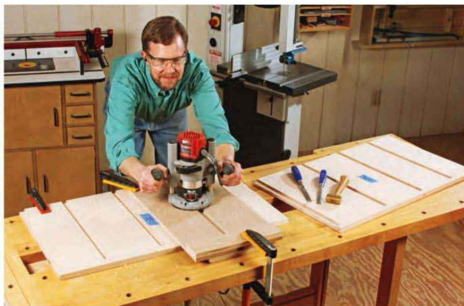
Matching side panel dadoes were easy to mill accurately with a slotted routing jig, rub collar and straight bit.
