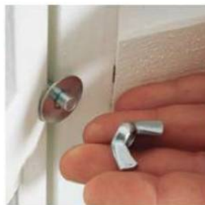
Trim pieces provided the gazebo with a more finished look. They also help to make the unit more stable. Place the trim pieces over the joints between the walls. Secure them from the inside with washers and wingnuts.
