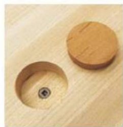
The inner three holes on the countertop house large 7" bolts with washers and nuts. The outer three holes are for 3" woodscrews (and, in fact, the center outer hole is just for looks).
