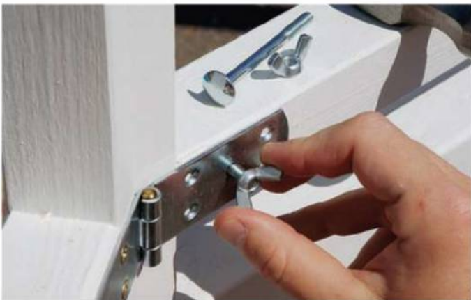
To connect the paired panels together, the author employed carriage bolts and wingnuts. All of the hardware should be galvanized.
