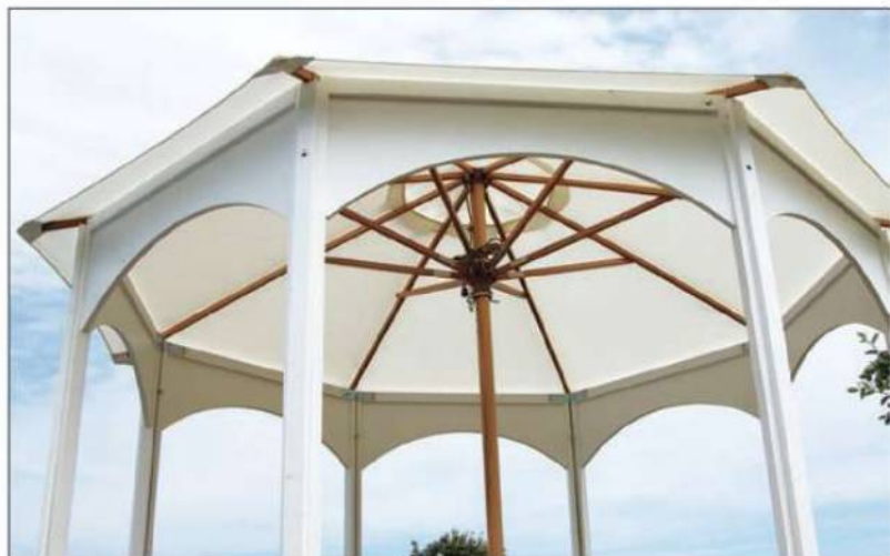
The author used a patio umbrella for the roof and hinges to join the eight wall panels, vastly simplifying his construction. Vertical trim hides the otherwise unsightly joints and also bolsters stability.
