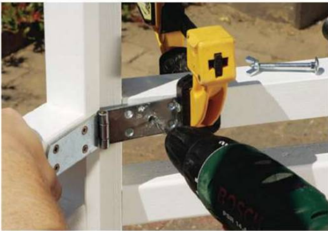
Using the clearance holes in hinge leaf he drilled previously, the author bored 5/16" pilot holes through the rails for the carriage bolts.
