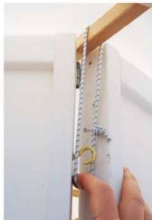
Eight 18" lengths of elastic cord looped over the umbrella's eight ribs help keep it in place even in high winds. The lines are tied together with square knots, and pulled onto the screw hooks.
