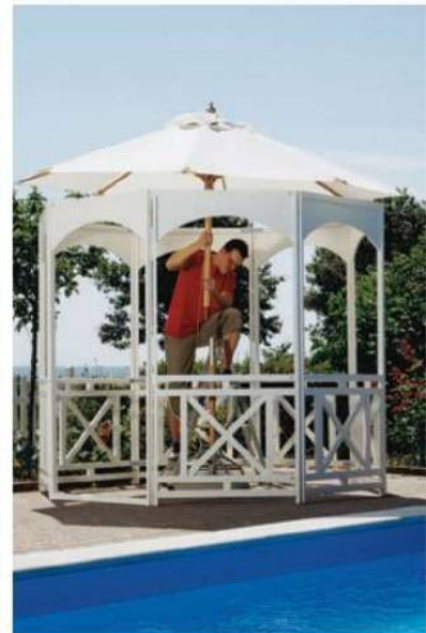
When the author was ready to raise the roof, he set the umbrella base exactly at the center of the gazebo, put the table in place and then set up the umbrella by coming down from the top.
