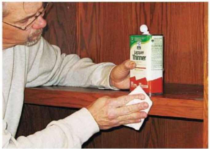
Before veneering, clean the cabinet surfaces completely. Follow behind the cleanup with a strong solvent of some sort to remove oils, polishes and years of grime that might interfere with your contact cement.
