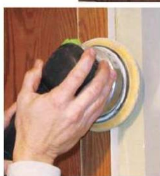
After applying the thin strips of maple veneer to the edges of the face frame, the author trimmed them flush to the wide face of the frame. He used both a block plane (above) and a power sander (left) to complete this task.
