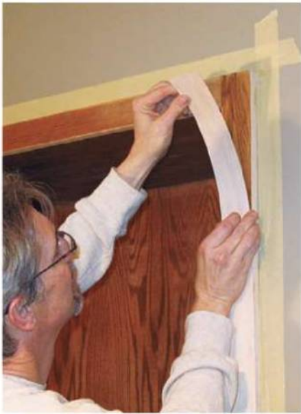
When applying the paper-backed maple veneer to the wide aspect of the face frame, the author started with the uprights and moved to the horizontal face frame pieces. This mimics traditional face frame joinery.
