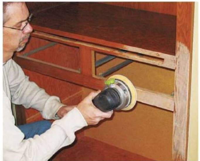
The author took a power sander to the front surface of the face frame. He did not try to remove the finish completely, but scuffed it up well. Following sanding, he wiped it down with a tack cloth.
