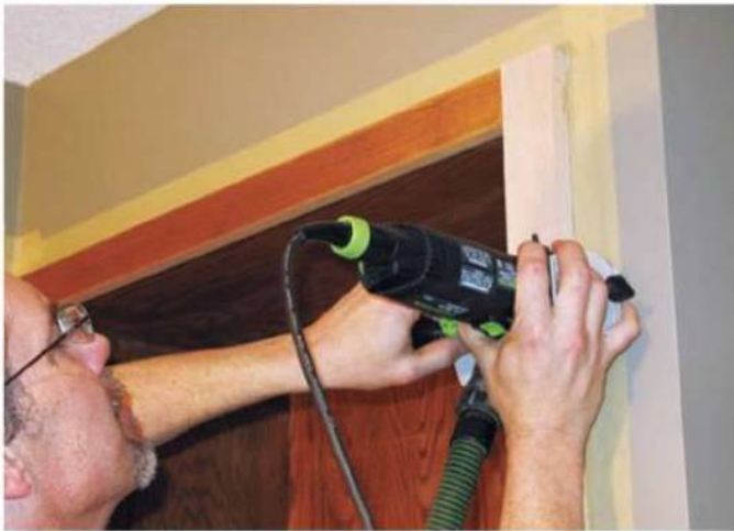
A laminate trimmer is a handy tool for this step of the process. The author followed behind the laminate trimmer by hand sanding the corners where the veneer pieces met.
