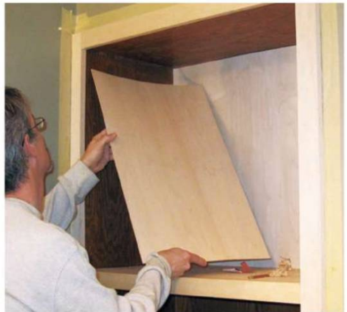
For the interior of the cabinet, the author switched from paper-backed veneer to 1/8" maple plywood. When faced with interior tight fits, the 1/8" plywood is much easier to manipulate. A couple of test fits, and it was ready to be applied.
