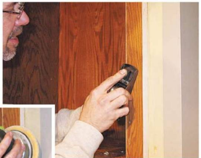
After applying the thin strips of maple veneer to the edges of the face frame, the author trimmed them flush to the wide face of the frame. He used both a block plane (above) and a power sander (left) to complete this task.
