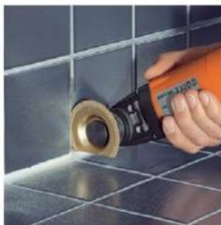
GRINDING: Since these tools cut in a linear motion, they offer precise grinding capability for grout and mortar removal.
