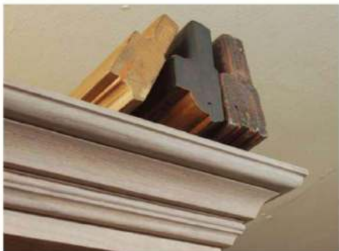
The crown molding is created from three separate pieces of shaped stock stacked to form the desired profile. The author builds the molding on the case so he can hide the nails that he uses to fight seasonal movement.
