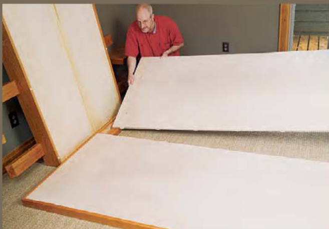
Set the platform plywood pieces in the frame. Place spacers under the joint between sheets to keep the edges from sagging. Then screw the plywood to the frame and lean the platform against a wall.
