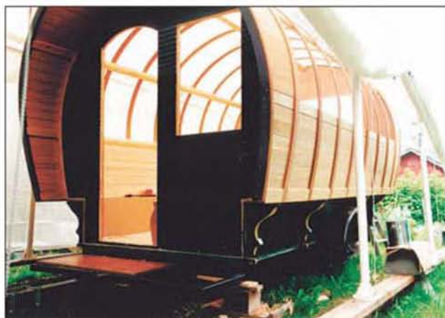
The author made the wagon roof from Egyptian treated canvas sailcloth laid over red cedar hoops, steam-bent over a form.
