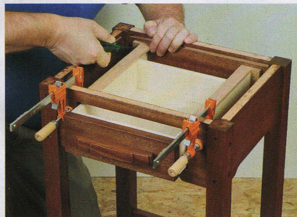
Mount the drawer support assemblies by first clamping them to the aprons so they keep the drawer centered and sliding smoothly, then screwing them in place.
