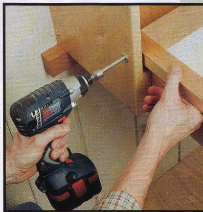
Drive four lag screws into two wall studs to install the cabinet. A temporary wall cleat allows you to place it accurately without a helper (right). Once the cabinet is up, mount the table by driving the pivot screws through pre-drilled pilot holes (above).
