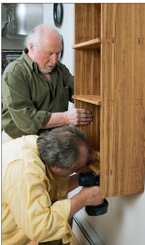
Mounting the bookcases to the wall is the final task. A cover strip top and bottom will hide the square drive stainless steel screws that David is driving home.
