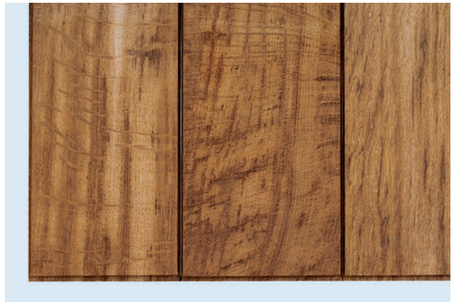
No aspect of the bookcase is ignored during the design process. Even the humble bookcase back is rich in detail. As shown here, the proportions of the back slats are also defined by "rebates" and shadows.
