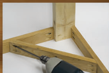
Assemble angle joints
