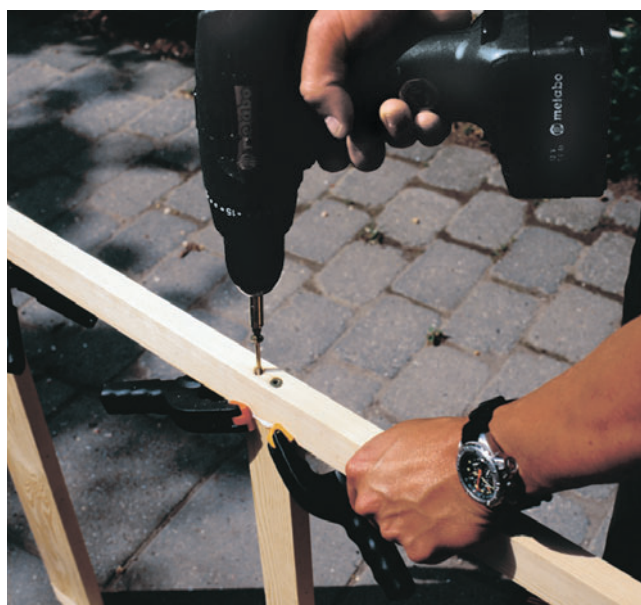
Join the wall panel members with glue and 3" wood screws. Use clamps to keep frame members flush while driving the screws. Allow the glue to cure.
