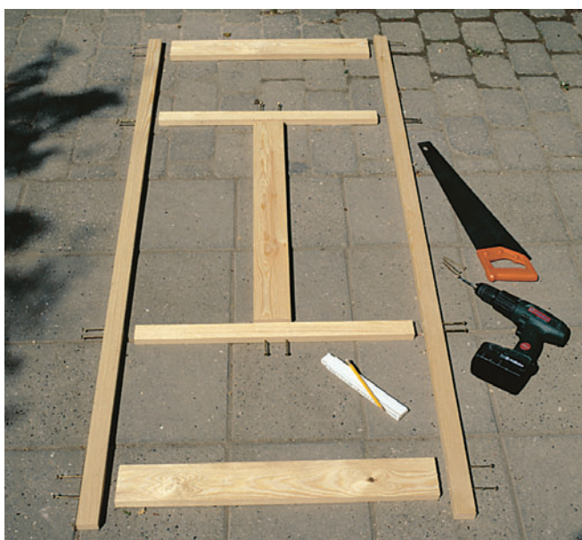
Cut out the parts for the two frames and lay them out on a large flat area, such as a patio or garage floor. Mark the screw holes and drill pilot holes. Take a few moments to work through the assembly process.
