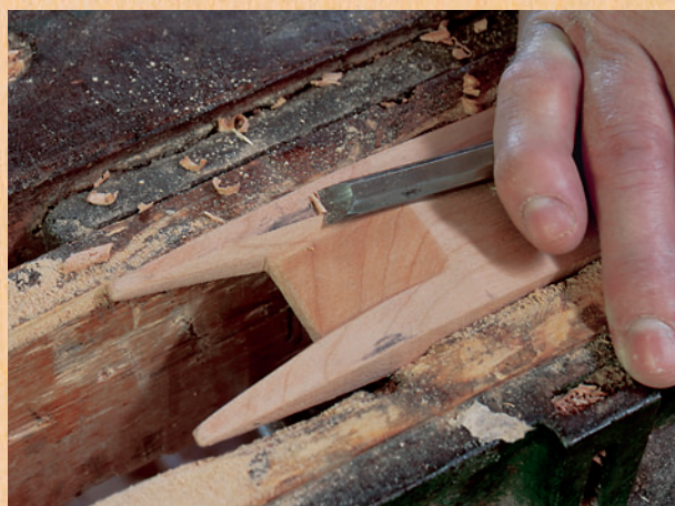
Figure 12: The pencil smudges from the previous step that you see in this photo indicate the location where final paring is required to fit the wedge into the assembly.
