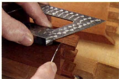
Position your marking knife in the line on the face of the workpiece, then slide the miter square to the knife.
