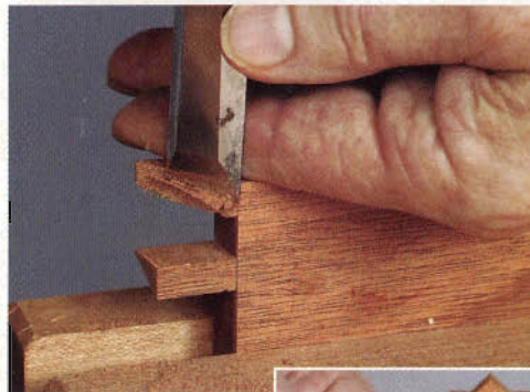
Establish the miter face by vertical paring for about 1/16", then set the pin piece in the vise at 45° and complete the miter using the small land as a guide.
