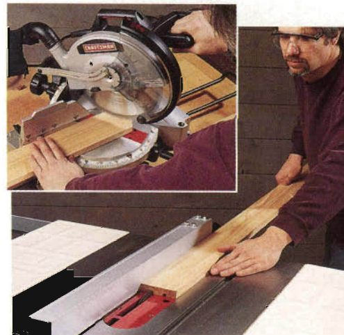
Form the dadoes on the sides before you cut them to final length. Use a power miter box saw to chop their 30° ends, as shown above.
