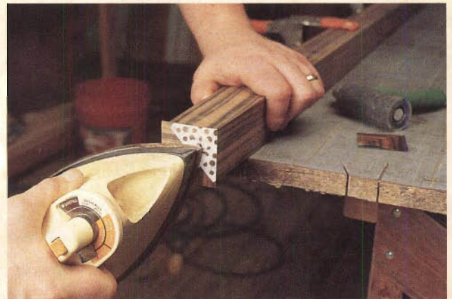
Ironing on his own pre-glued veneer is a technique the author used to ensure perfect placement. He used this method on the leg caps (shown above), the long aspect of the legs and the cabinet's face frame members. Large panels are vacuum bagged.
