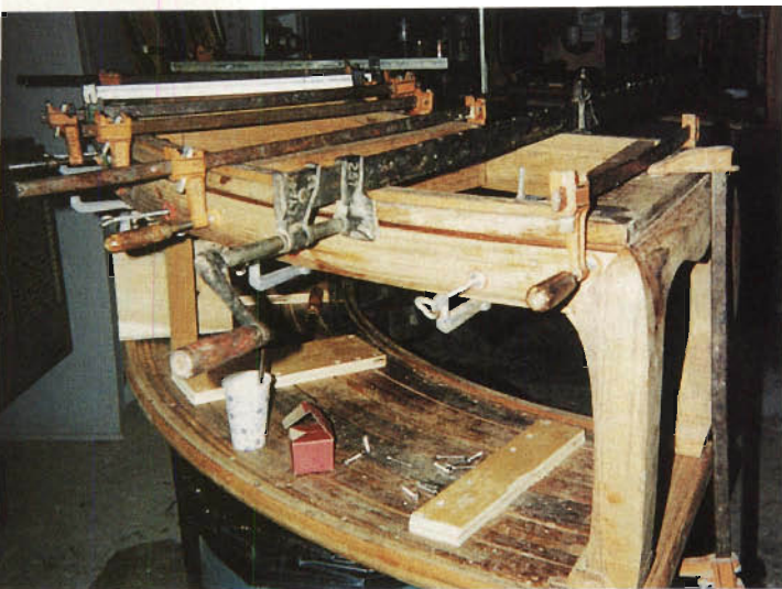
Using the Top as a Template: Glue-up and assembly of the benches' internal frame was done while it sat on top of the completed seat plank subassembly. This proximity helped to ensure that the construction process moved along smoothly.
