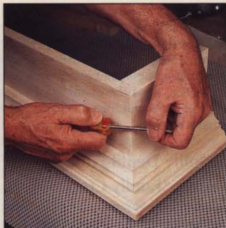
Photo F: To close any gaps on fascia miters, daub glue into the crack, then roll the corner with a screwdriver or burnisher.
