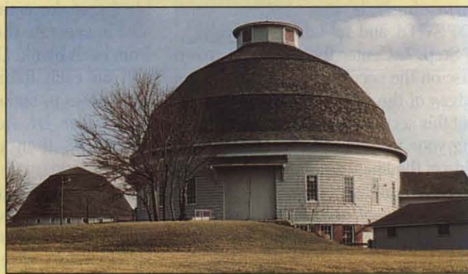
The round barn offered economical construction, convenient livestock feeding, and resistance to strong winds. These barns, built by the University of Illinois between 1907 and 1913, served as model facilities for a demonstration dairy farm.
