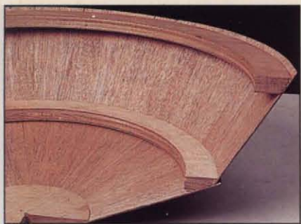
Photo B: This view of the assembled roof shows the beveled, cut-away profiles of the rings and crown disc.
