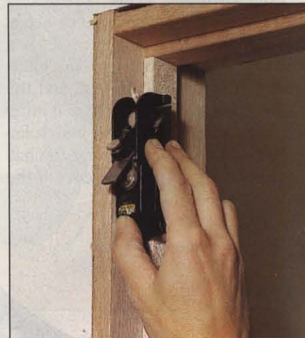
Photo G: The bullnose plane is the perfect tool for trimming door jambs and other tight spots.
