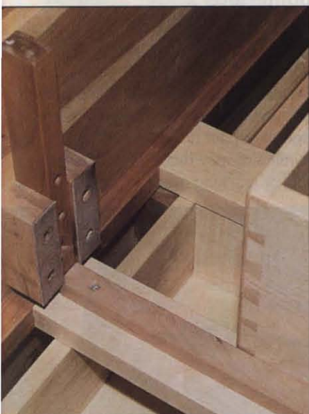
Photo G: Leather-faced drawer stops mounted on each side of the stanchion limit drawer movement.
