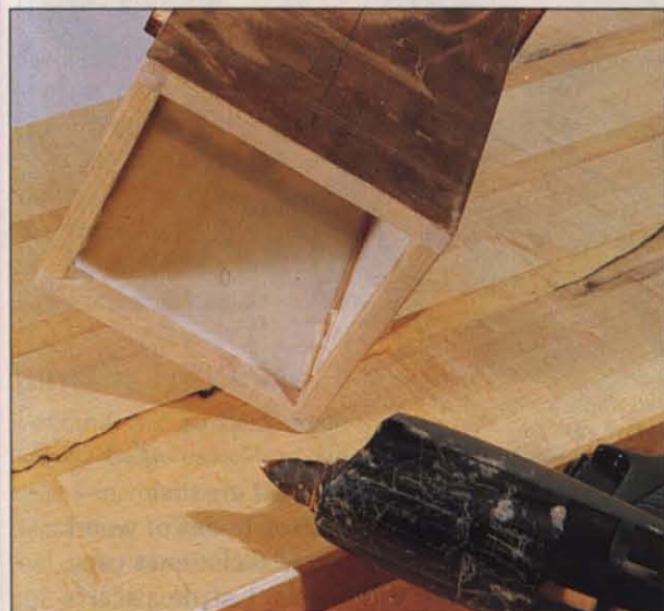
Photo A: A bead of hotmelt glue along the inside edge of each pane and post tacks the panes in the frames so you can safely caulk the outside edges.
