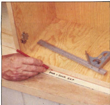
Photo A: To crown a cabinet with complex molding, author first makes a full-scale template of the cabinet top. If the molding must overhang an overlaid door, remember to allow for it.
