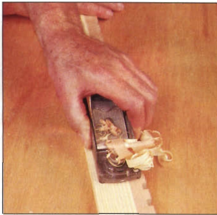
Photo H: After gluing dentil stock to slightly thicker pine backing strip, plane backing flush. Note that backing strip will be hidden by first and third layers after assembly.
