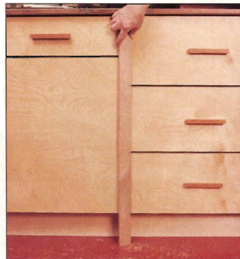
Photo A: A story stick precisely locates the position of parts and reduces the chances of misreading a measuring tape.
