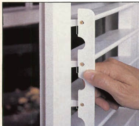
Photo E: Shutter openers are attached with screws for more durable construction and mounted to the side for a cleaner look.
