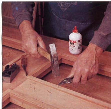
Photo H: Glue and nail outside molding to frame using type II water-resistant glue (or polyurethane glue sparingly, as author did). Pilot-drill holes, drive brads, then set brads and fill holes.
