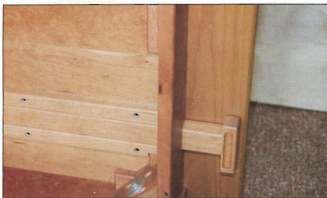
Photo B: The underside of the table. Note how the leaf support slides freely between the two leaf support guides attached to the top. Author also used wooden corner blocks to attach legs to aprons.
