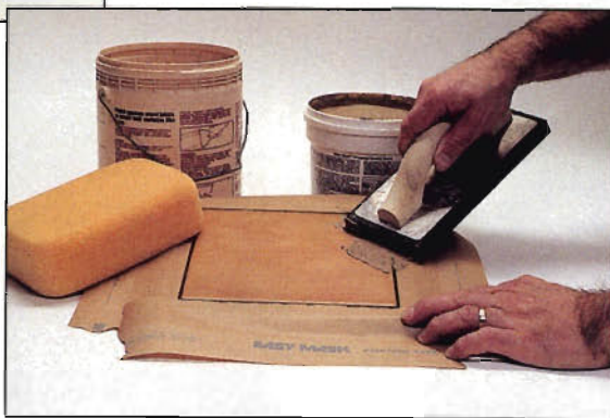
Photo J: Using a rubber float to grout the tile simplifies this phase of the project and ensures good results.
