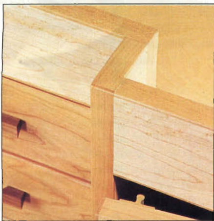
Photo D: Outer front panels overlap dividers, which in turn overlap center front panel. Note edge banding on panels and door.
