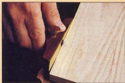
Photo K: Using a marking gauge, lay out the depth of the hinge gain.
