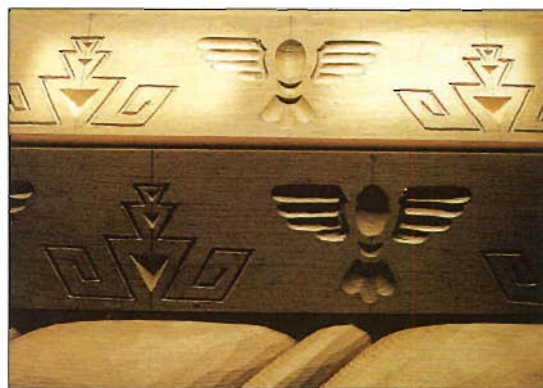
Photo C: Architectural panels and rope molding. Sugar pine with stain. La Posada Hotel restoration, Albuquerque.
