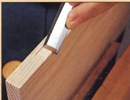
Photo O: Make a series of cuts on the face of the gain, holding the chisel bevel side up at an angle of 30°.
