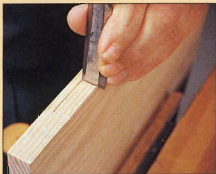
Photo N: Square the shoulder of the gain using a chisel.
