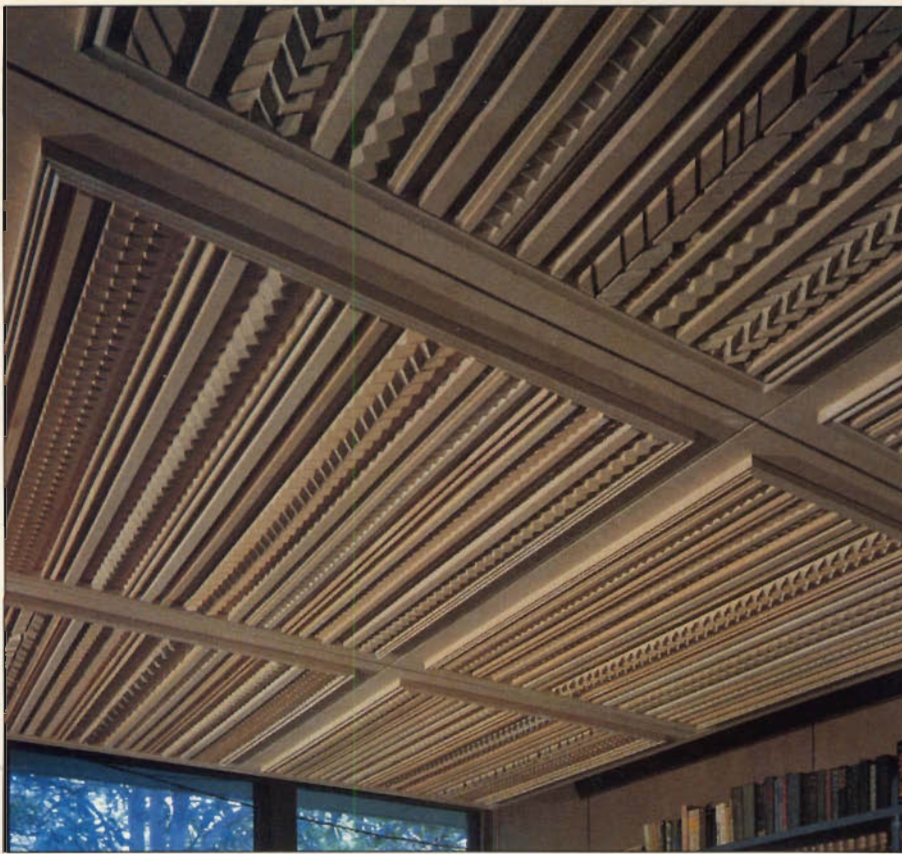
Assembled from numerous narrow carved boards, this 11 1/2 x 15' ceiling must have kept Ford and his workers busy for weeks.
