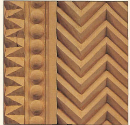
Assembled from numerous narrow carved boards, this 11 1/2 x 15' ceiling must have kept Ford and his workers busy for weeks.
