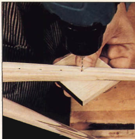
Photo J: To drill net holes, start with a \frac{5}{64} " bit for angle correction, then enlarge with a \frac{1}{8} " bit.
