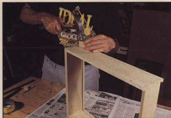
Photo R After pushing the joints together by hand, you can drive the tails home with a few sharp raps on a narrow hardwood block.
