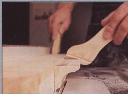
Photo J Elevate the saw blade, and cut a shallow kerf along the top edge of the cove to break the cove's edge.
