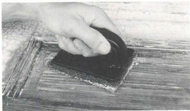
You can't use steel wool or metal scrapers with the dibasic ester safe strippers; 3M offers this handy stripping tool with replaceable plastic scouring pads.
