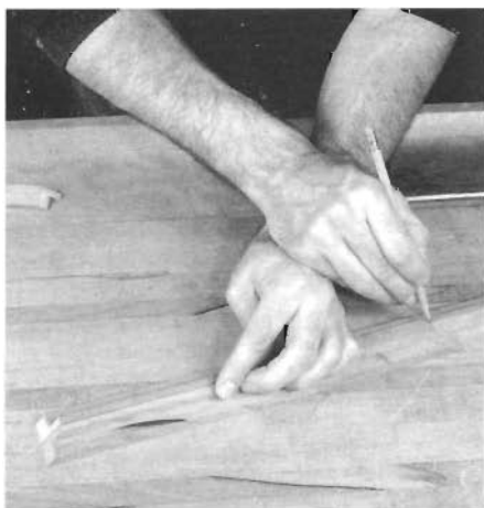
Photo 4: For identical sides, cut the first, then mark the length of the second from it.
