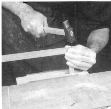
Photo 7: Continue holding the joint together and drive in the nails.
