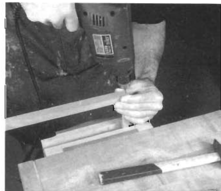
Photo 6: Hold the glued miter joint together with one hand while you bore pilot holes for the nails with the other.
