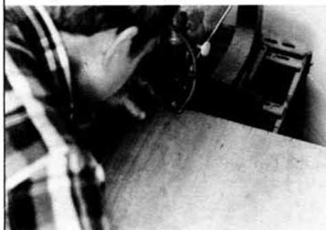
A jig saw is used to cut just inside the scribed line. A small dovetail saw can also be used here.
