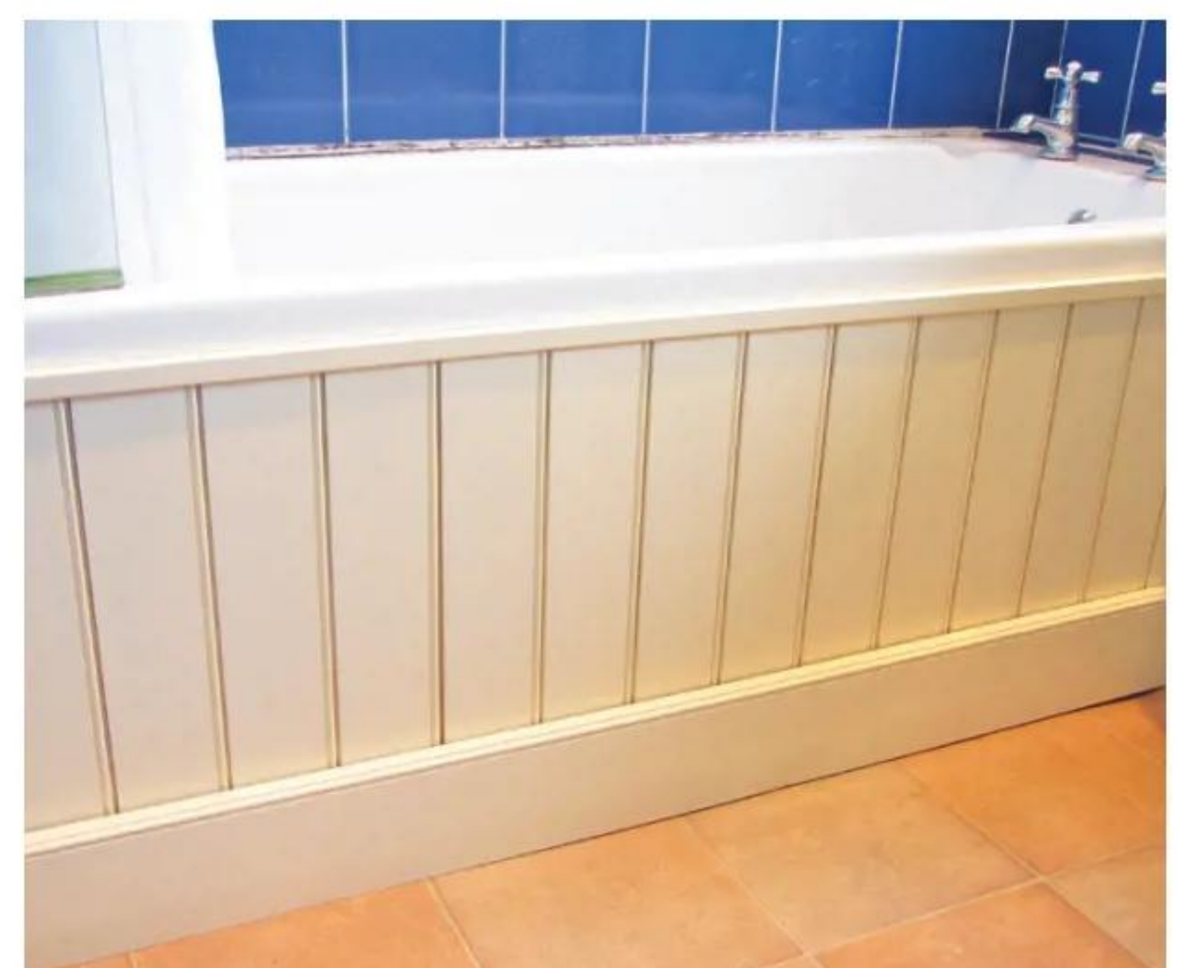
24 The finished panelling is a big improvement and gives the bathroom a more informal feel ✕
