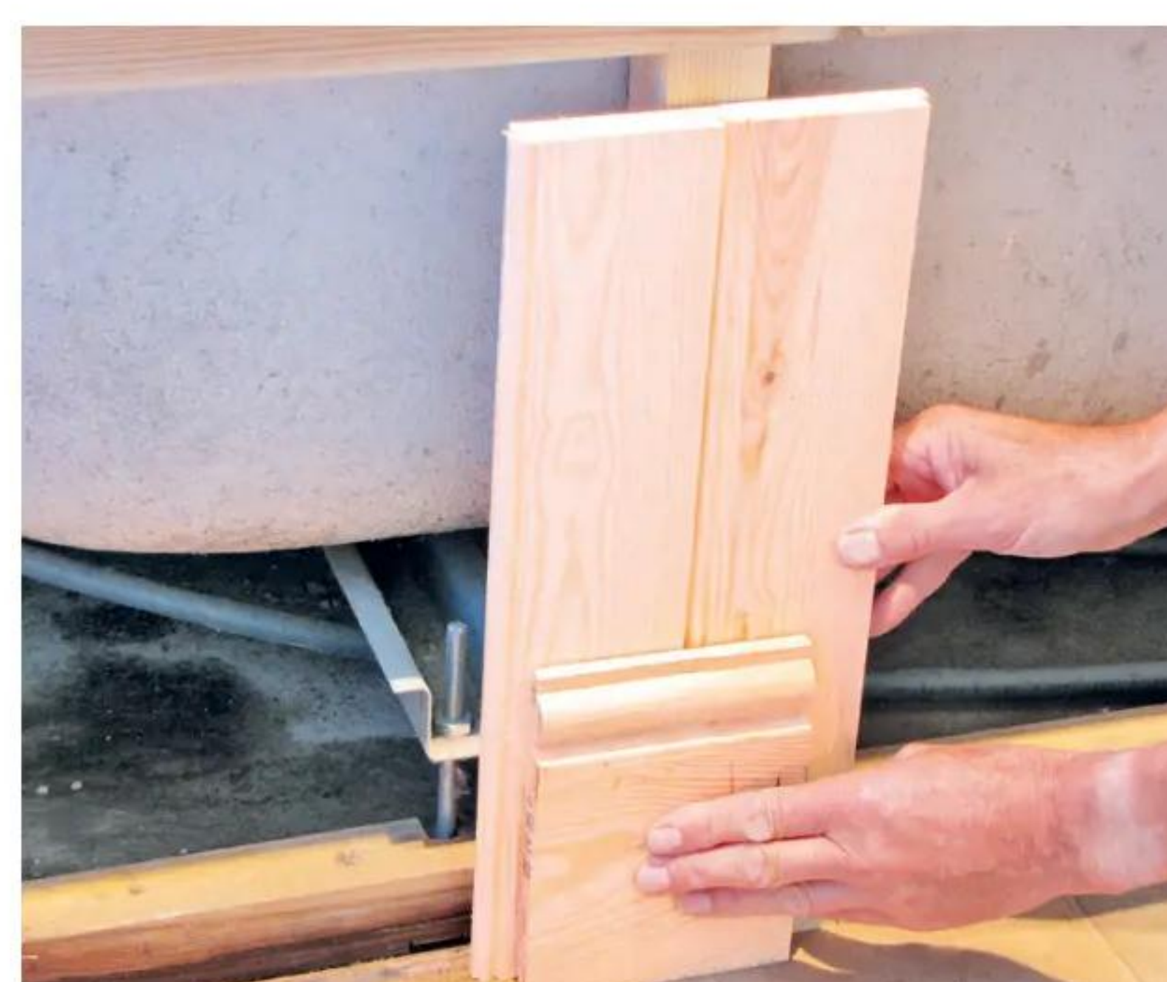
12 Decide on skirting height using an offcut held against the boards; this looks too deep
