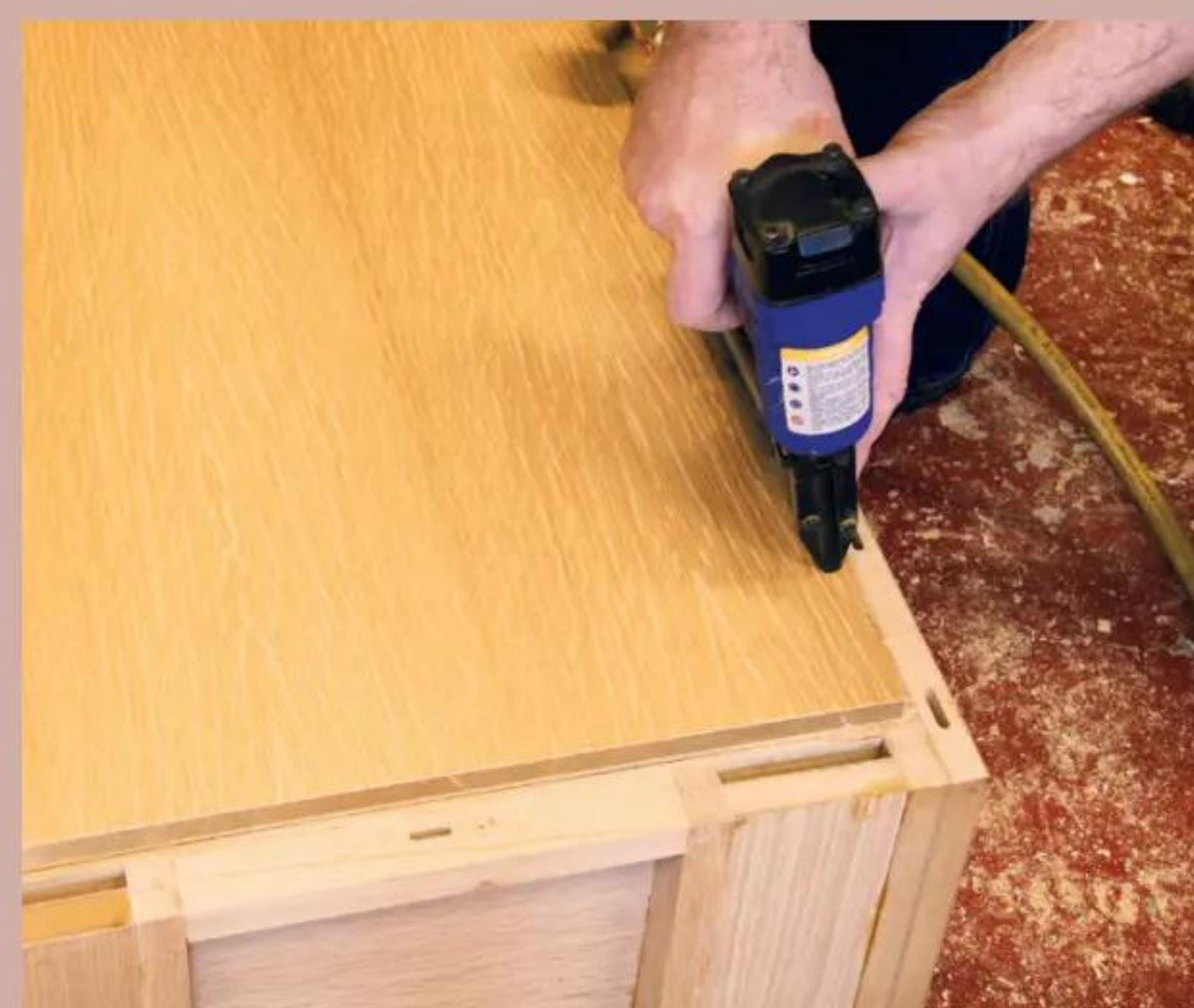
19 The rear panel was held in place with brads
