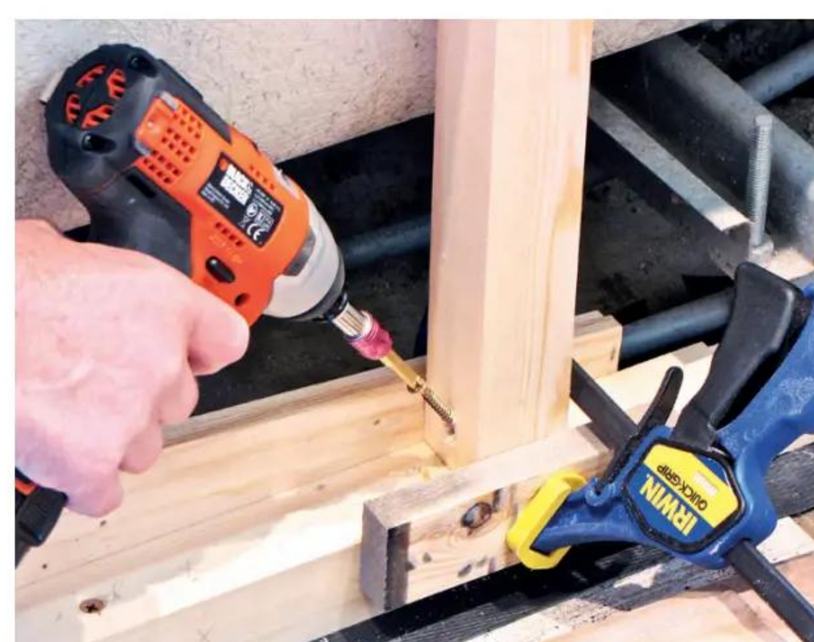
6 Cramp ends of the uprights to prevent slipping, then drill and screw these securely to the bottom rail
