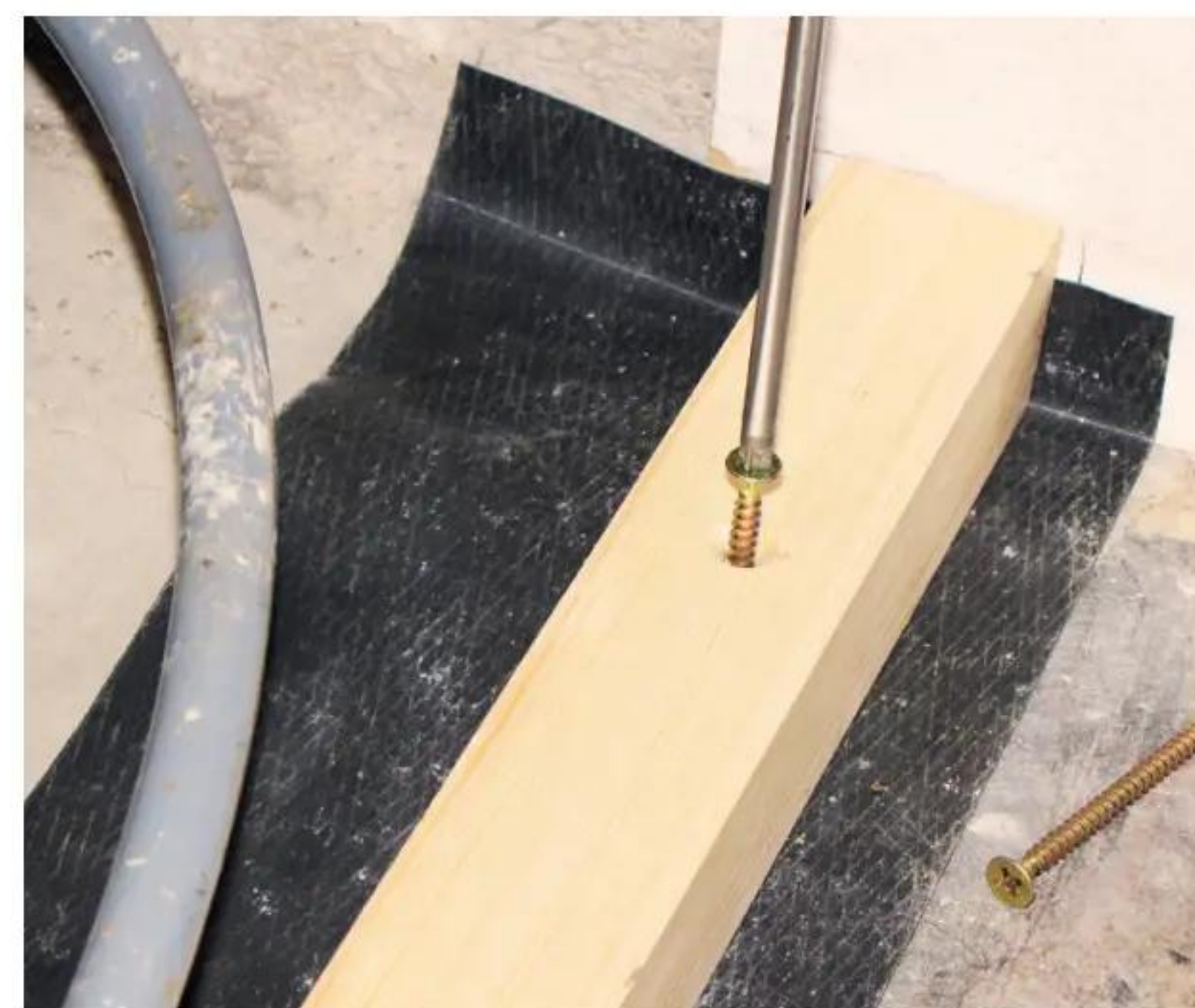
3 Cut the frame's bottom rail to length; drill and countersink, insert plugs in concrete and screw to the floor
