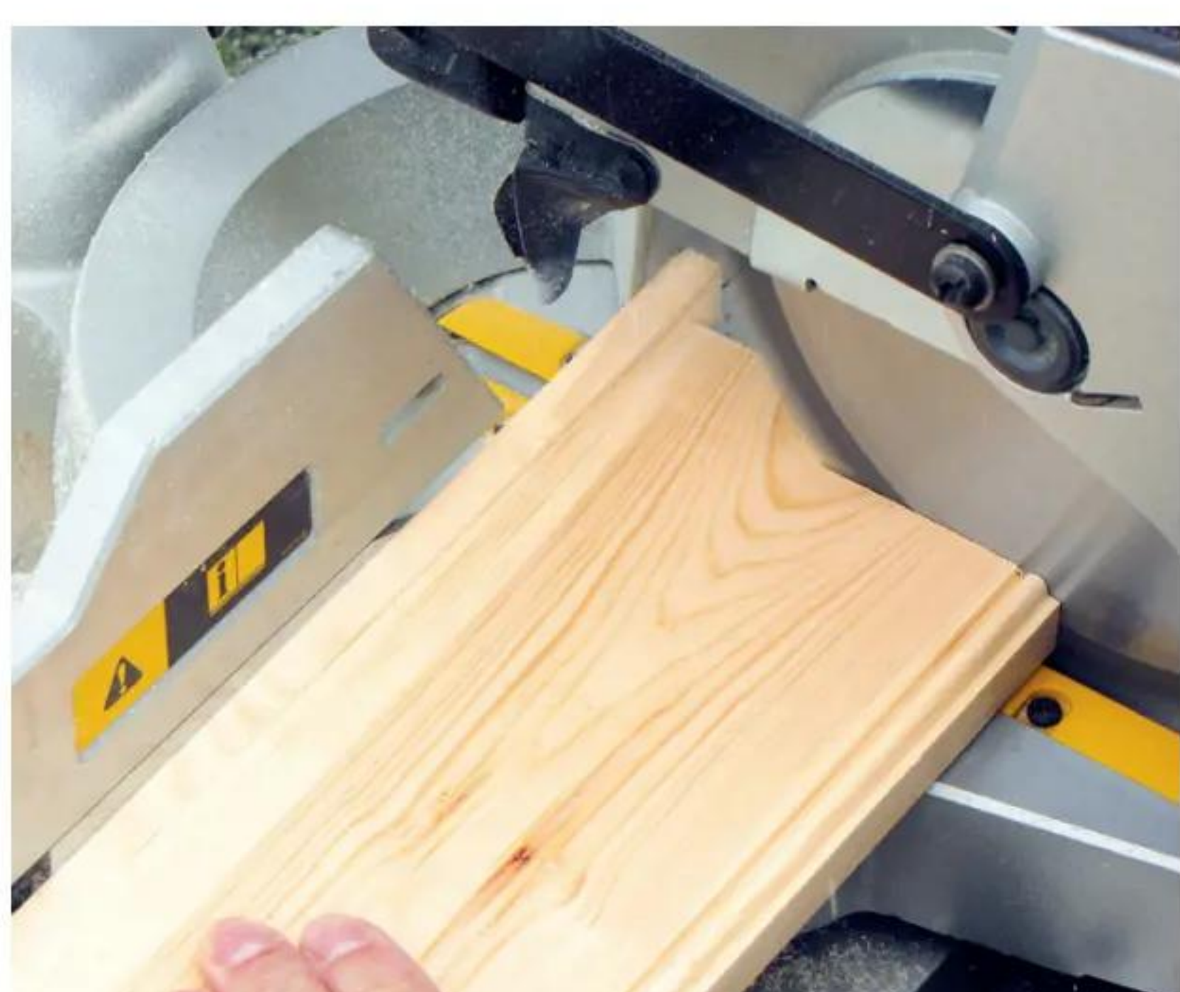
10 Measure finished height of boards and saw to length; an offcut at the rear prevents breakout
