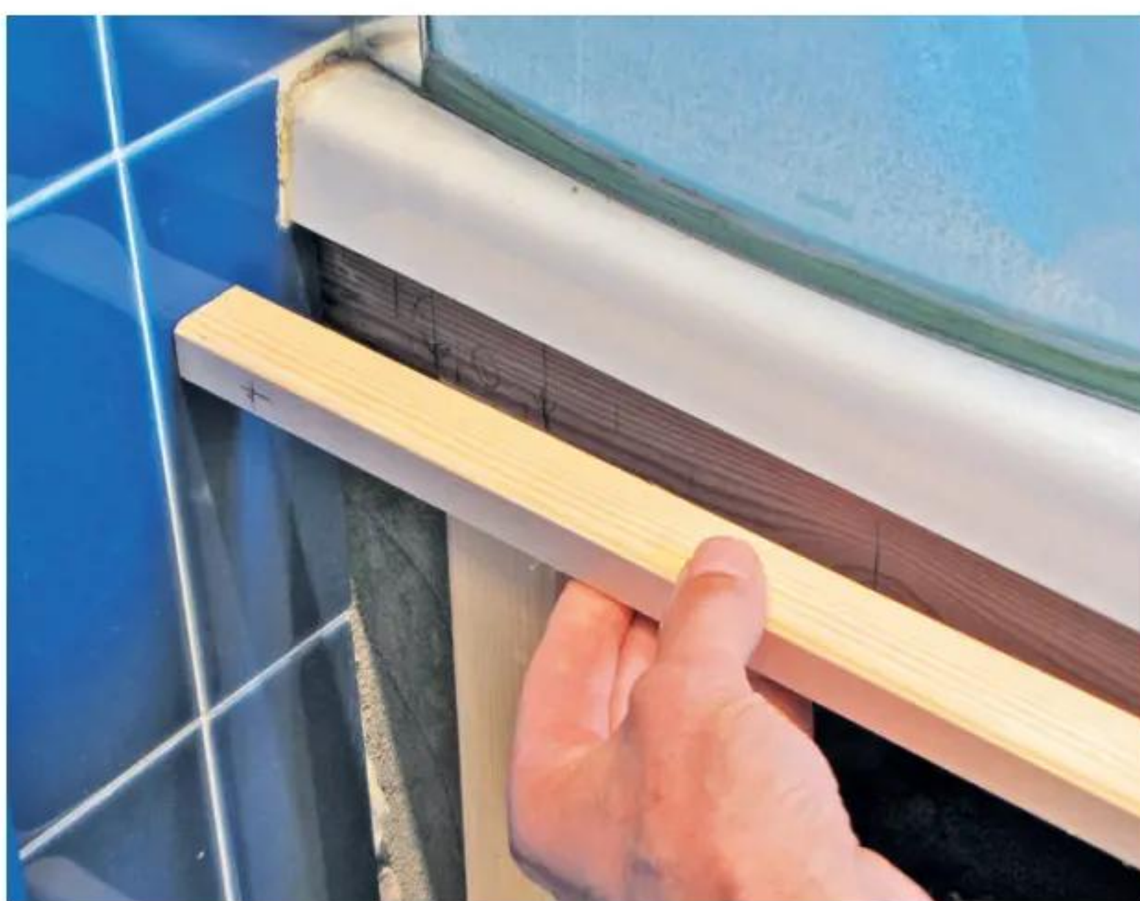
16 Cut capping to length and chamfer the edges; this sits underneath the bath edge and is nailed in place
