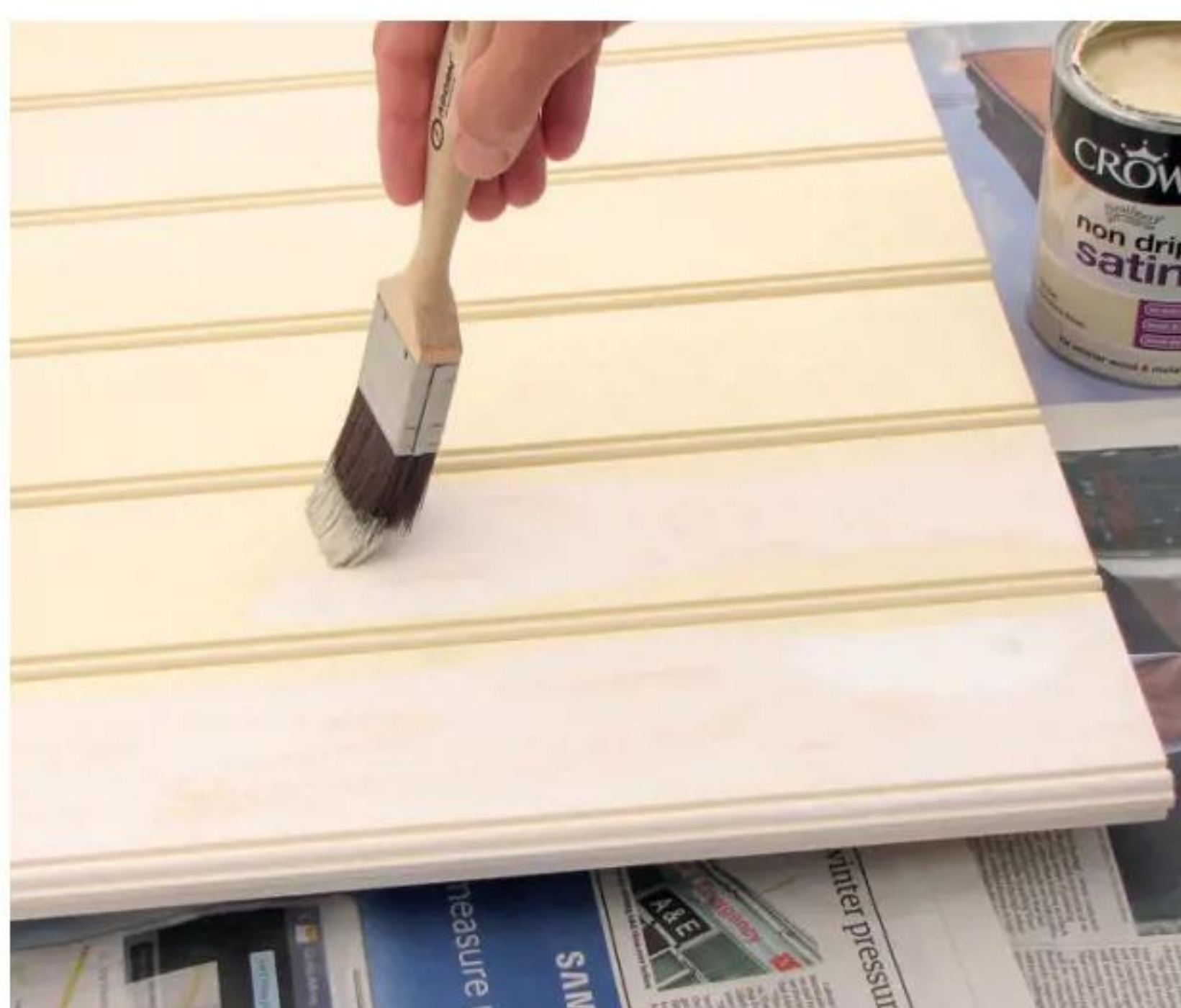
23 Mask off the bath edge, prime bare wood and brush on two coats of suitable satin paint
