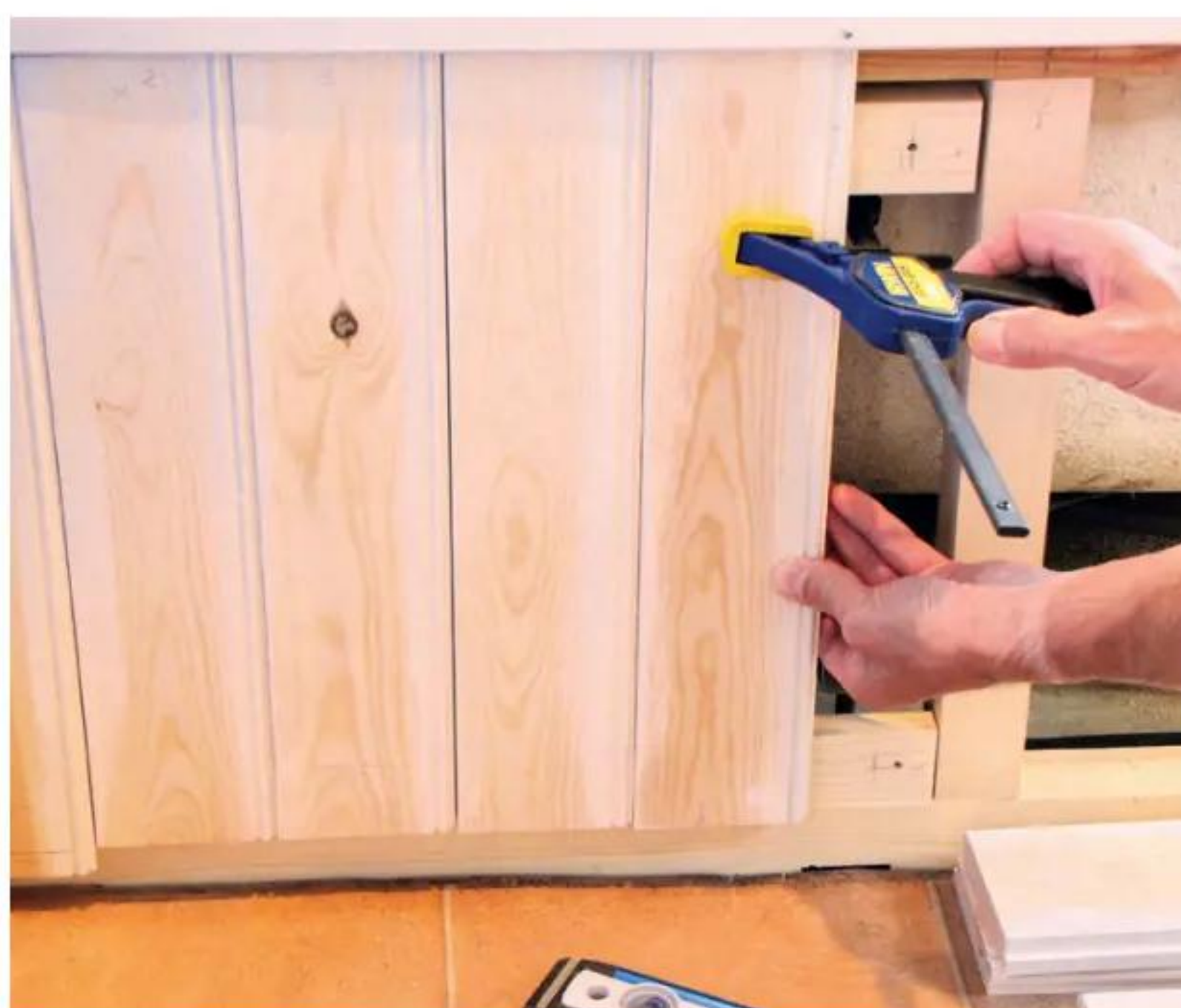
20 Continue along the bath side, cramping each board before screwing to the batten
