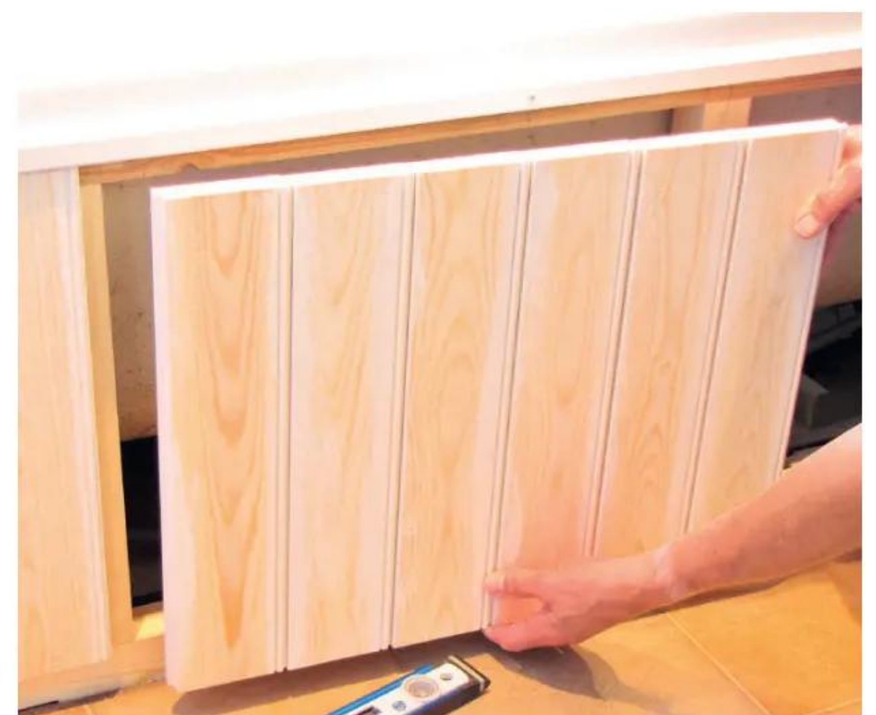
21 Made up of three separate panels, each one can be lifted out of the framework for ease of access
