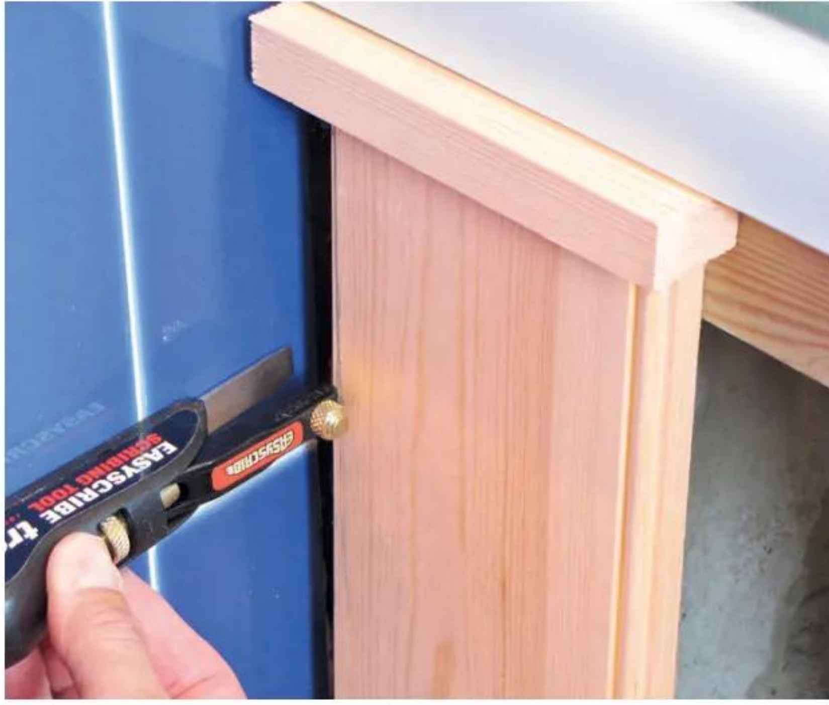
13 If walls are uneven, scribe first board with the Trend Easyscribe tool; ensure the board is plumb
