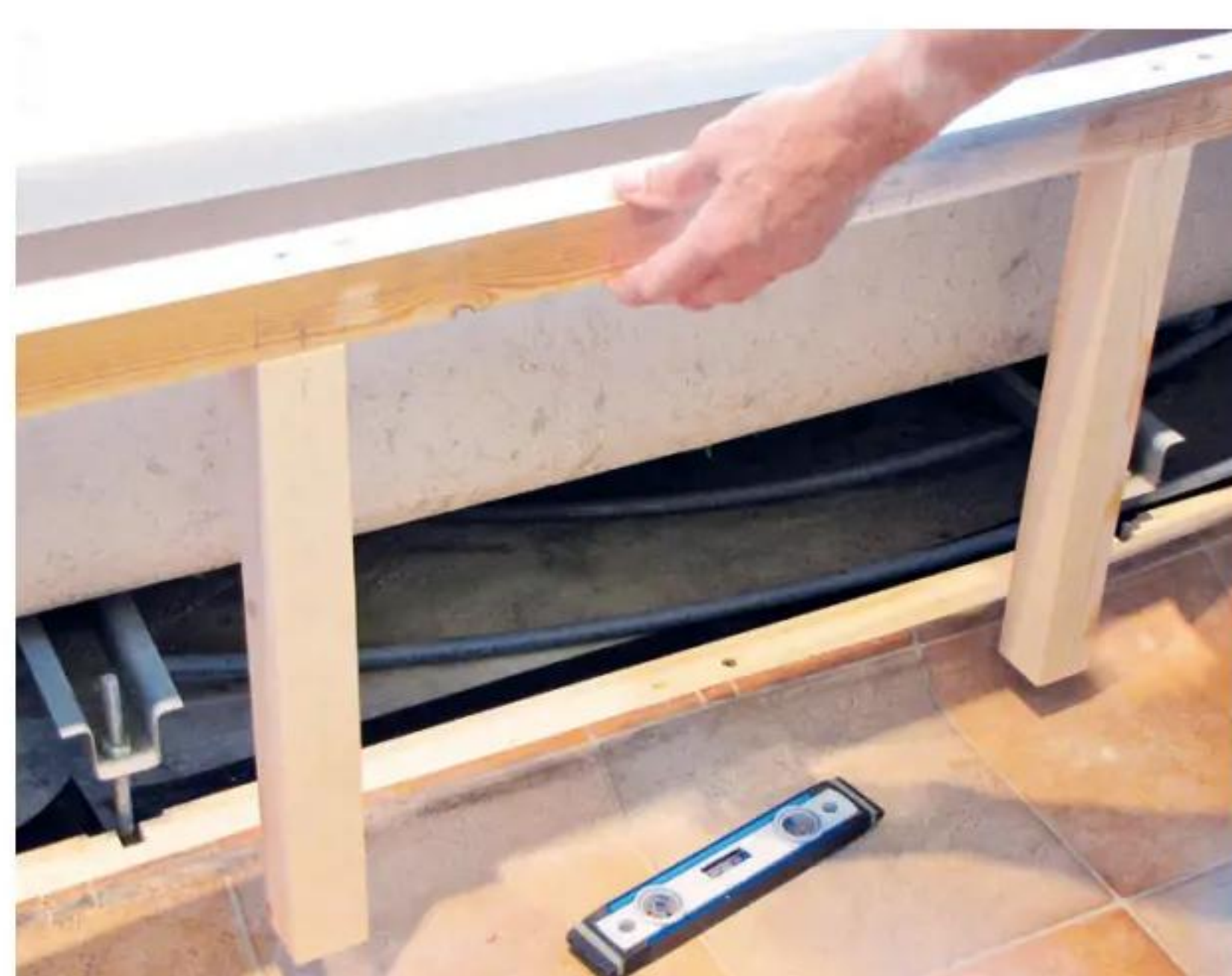
5 Position framework in place under the bath's edge; tap with a hammer, but be careful not to overdo it
