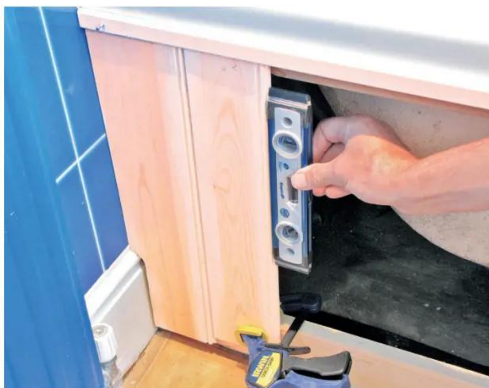
17 Position first two boards against the framework and check with a level; cramp to the lower batten
