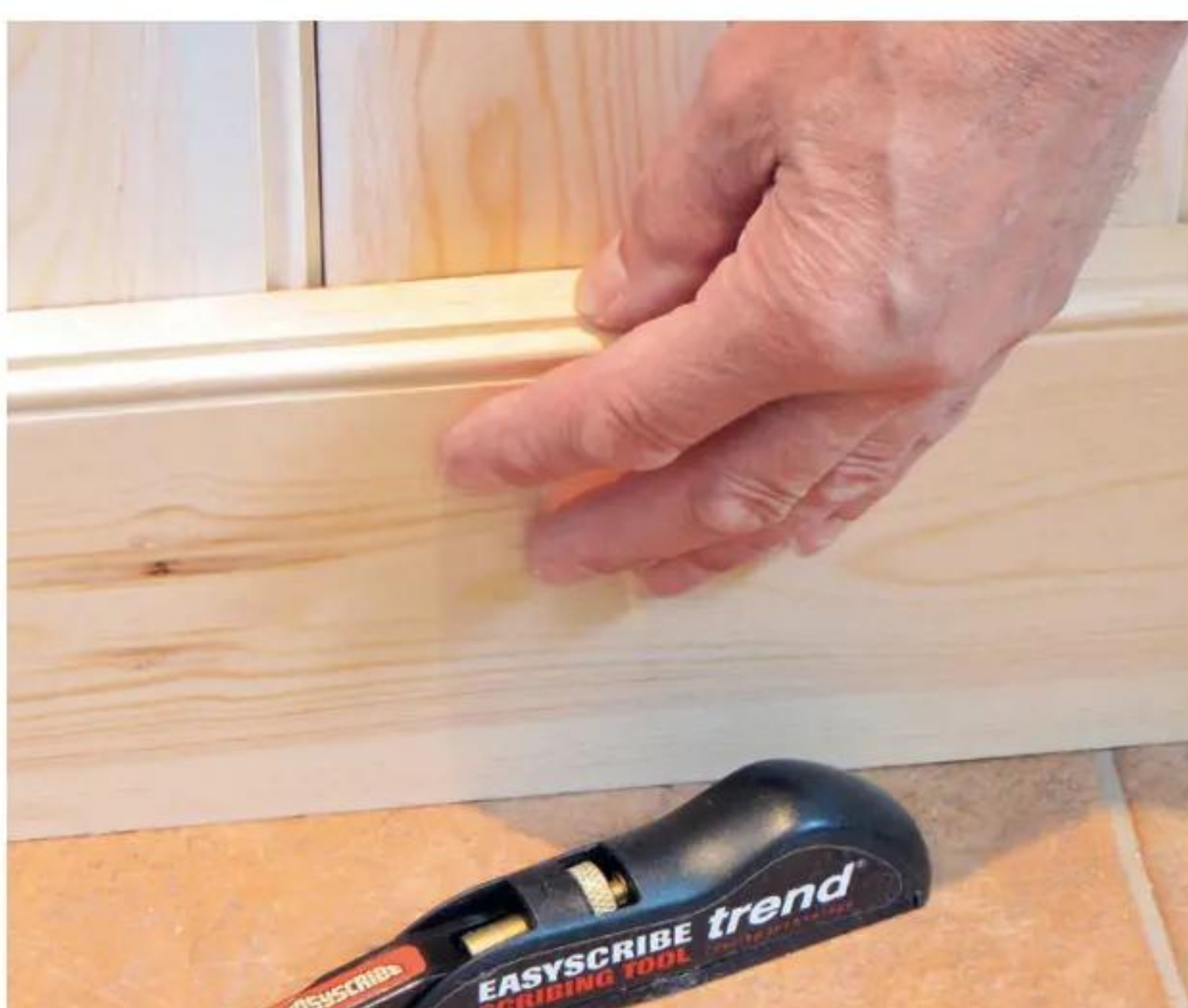
22 Cut skirting to length, scribing ends if necessary; rout a beaded profile along the top edge
