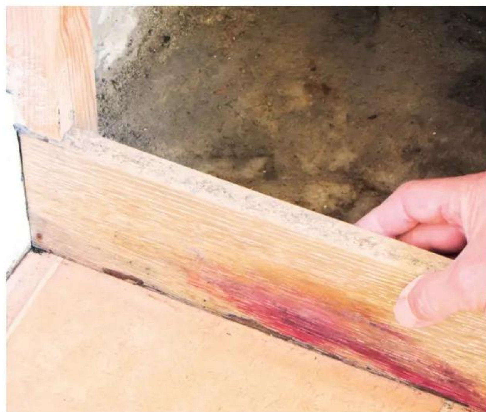
2 Remove the kick board and cut away old timber; renew sealant around shower and bath if suspect
