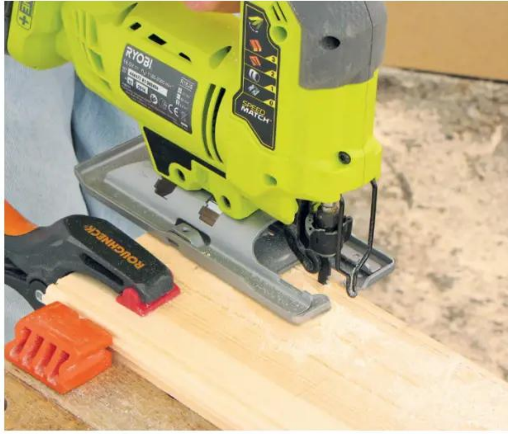
14 Cut along the scribe line with a jigsaw; hold board against wall and trim the edge if required
