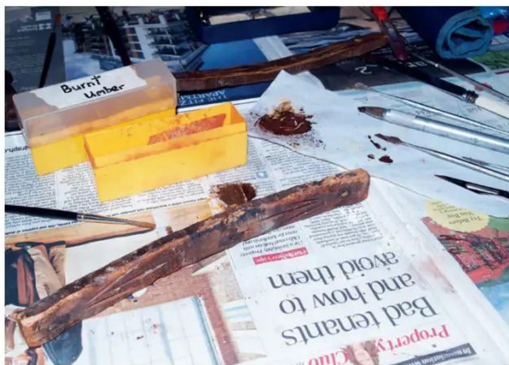
6 The epoxy was colour-matched with earth pigments to match the surrounding surface
