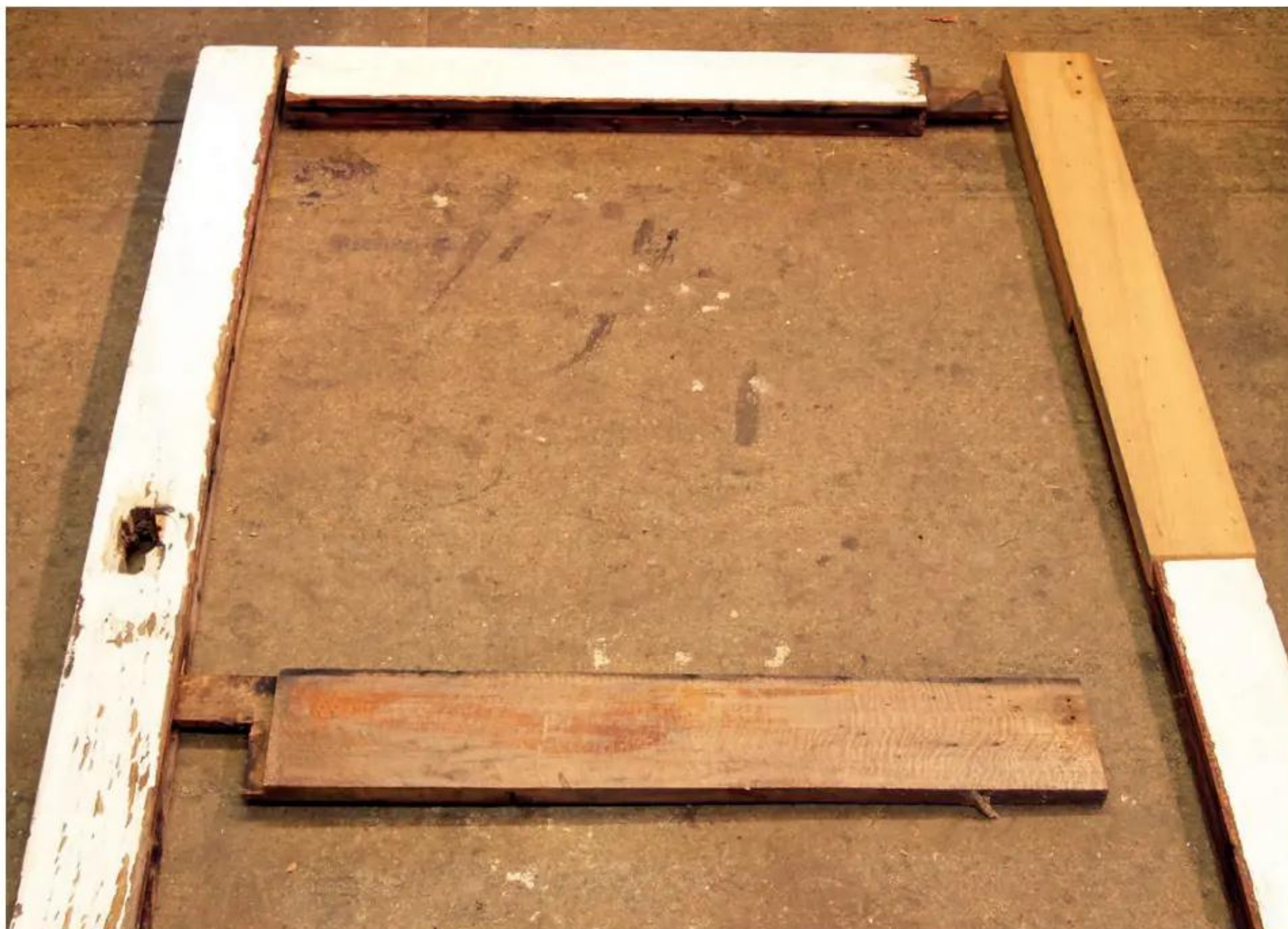
1 The door timbers disassembled
