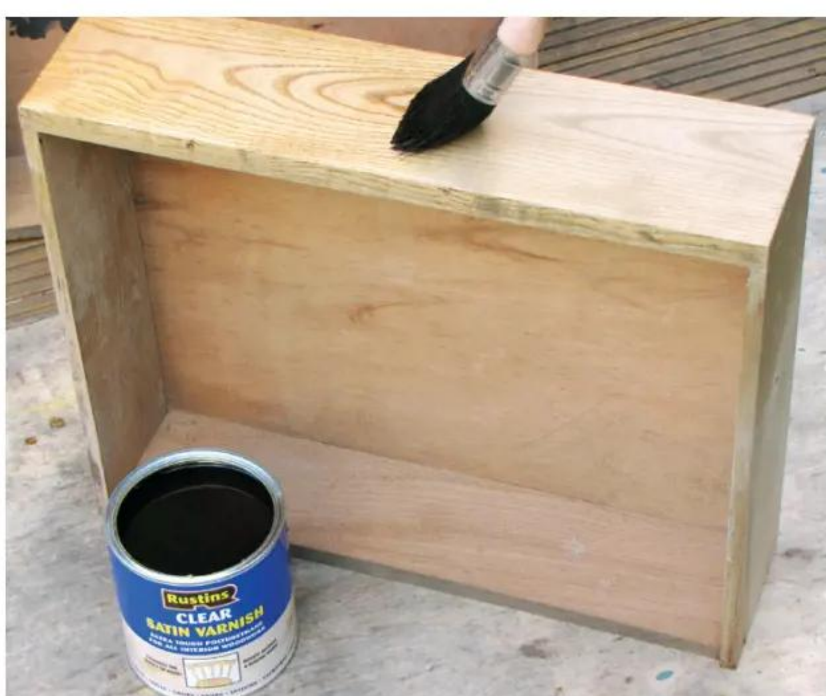
12 Brush on two coats of suitable satin or matt varnish, thinning the first one with white spirit if necessary
