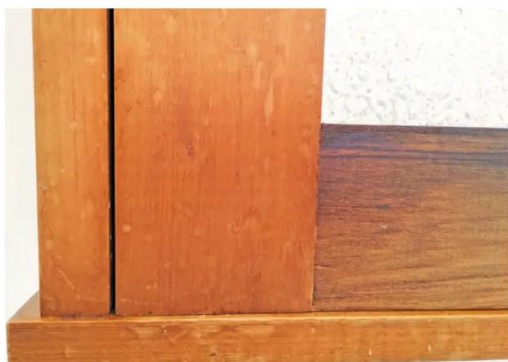
Water stained Paraná pine cabinet
