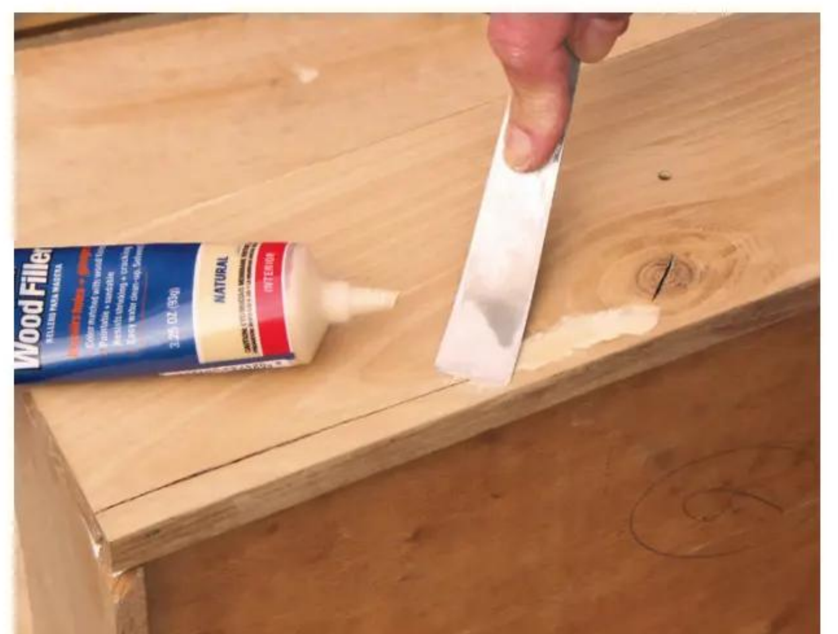
8 Fill any cracks or blemishes with matching filler and sand back when dry; this may need tinting later
