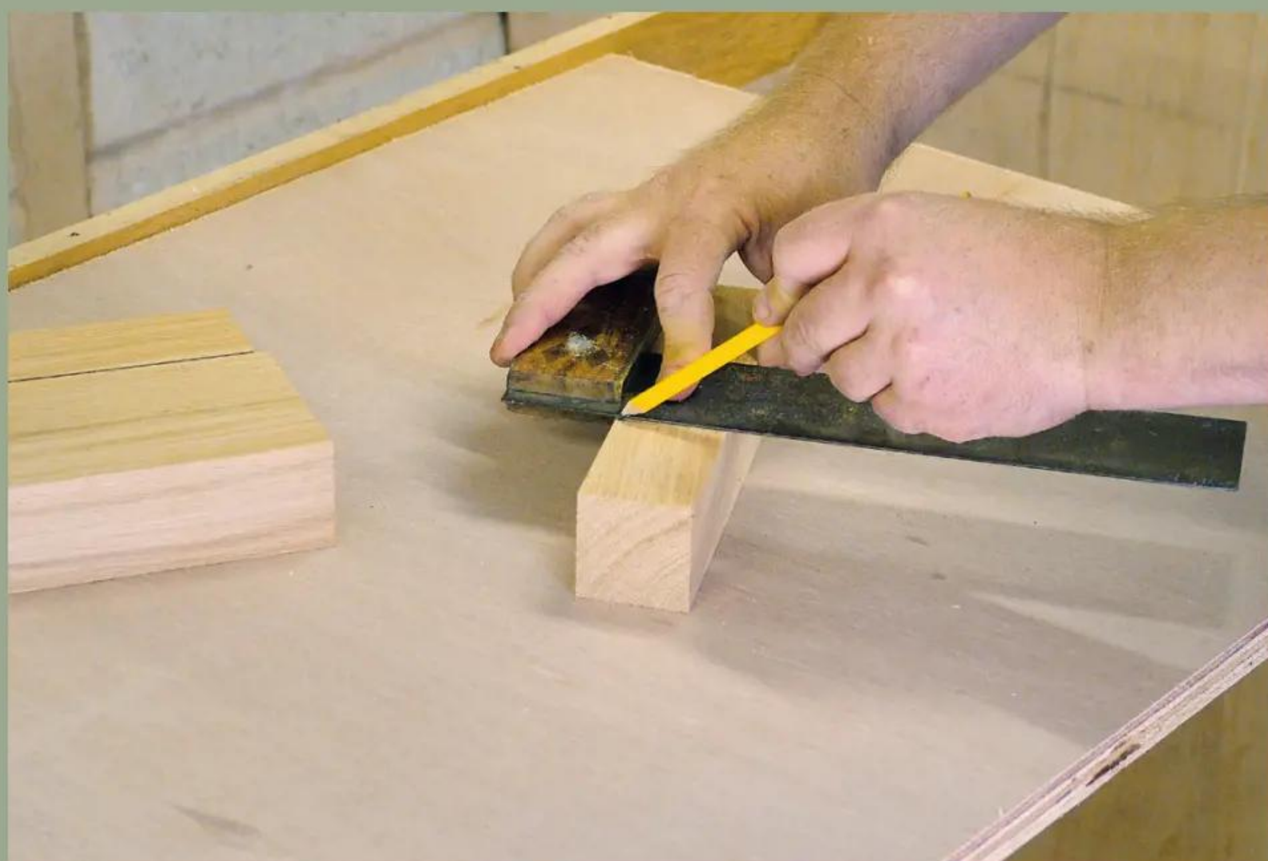
6 Measure 63mm from one end and square a line round all four faces
