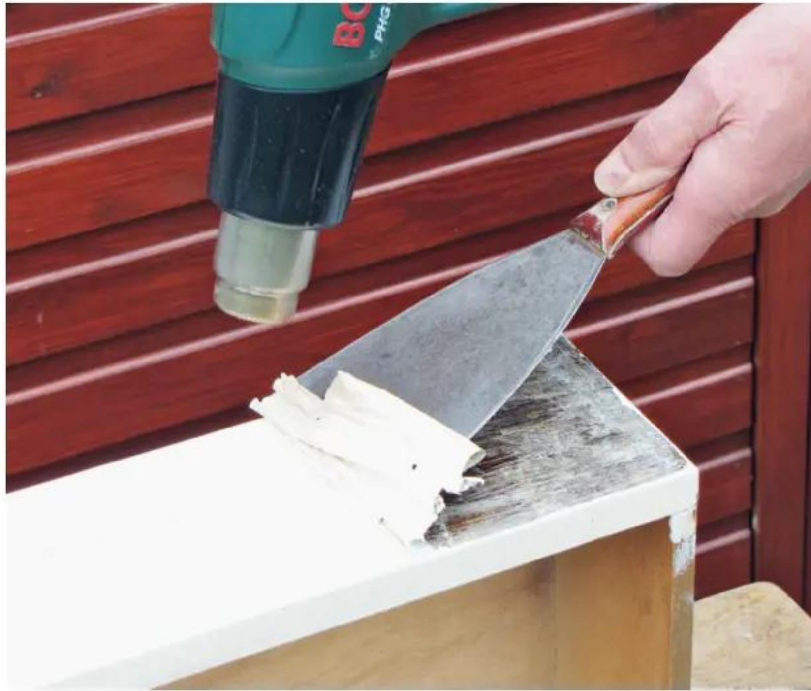
4 A heat gun used with a shave hook or stripping knife is the fastest way to remove several layers of paint
