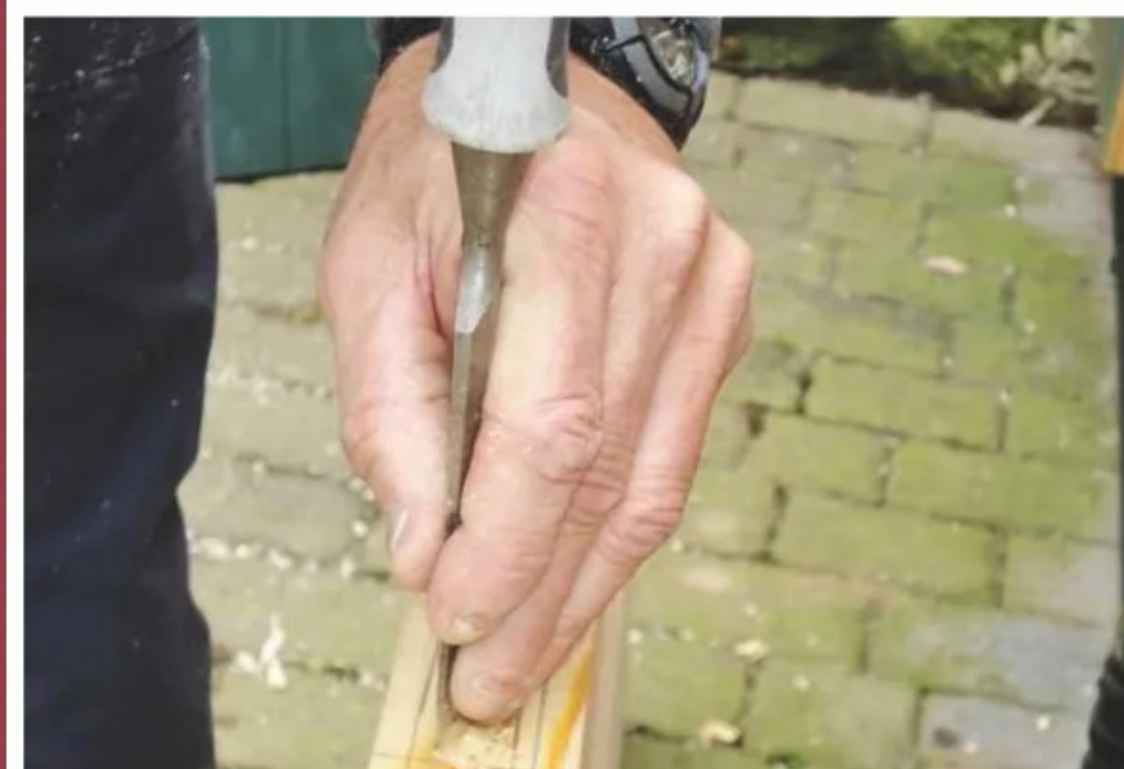
3 ... which was then cleaned up with a chisel
