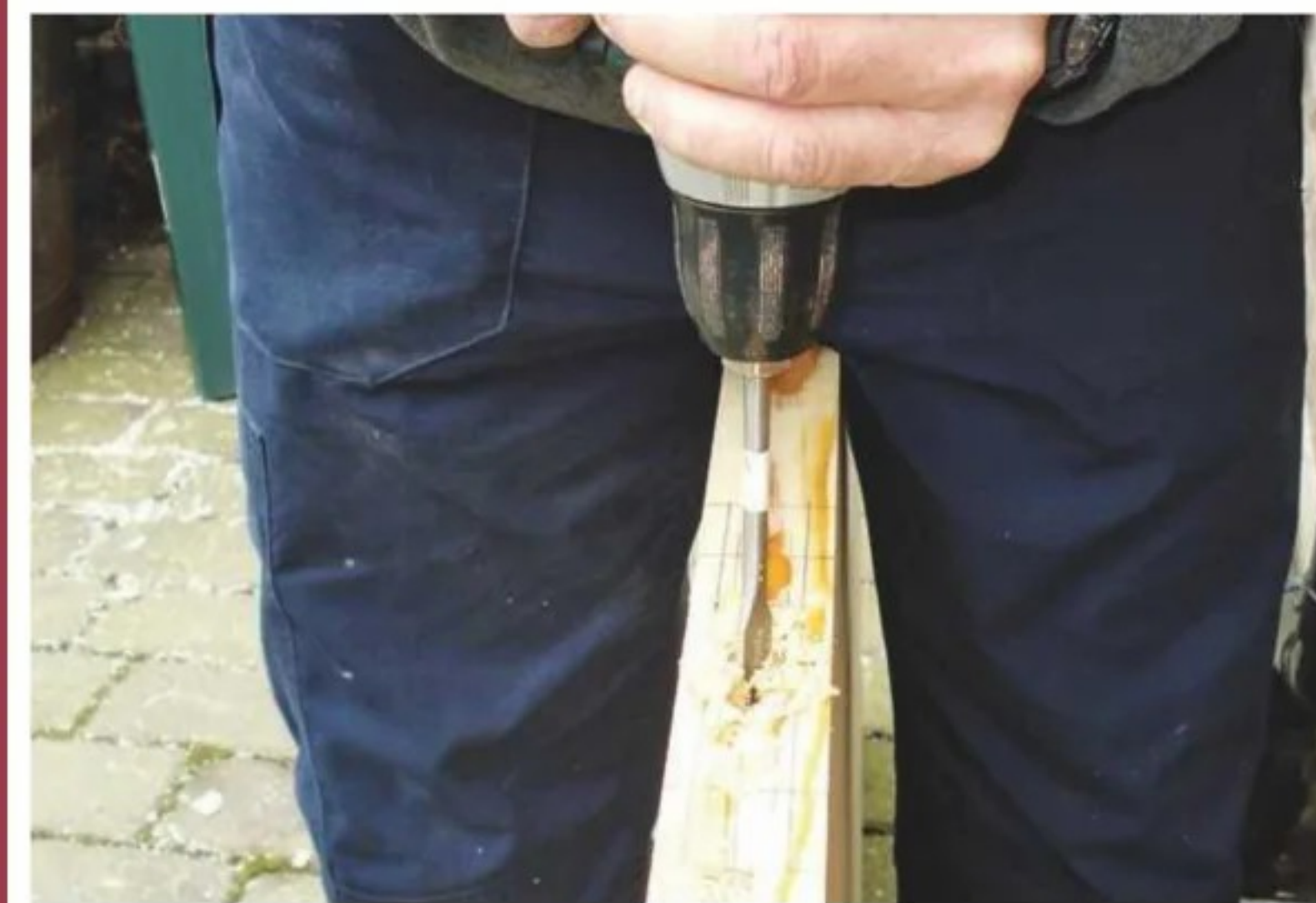
2 Using a flat bit in the cordless drill to cut one of the mortises...
