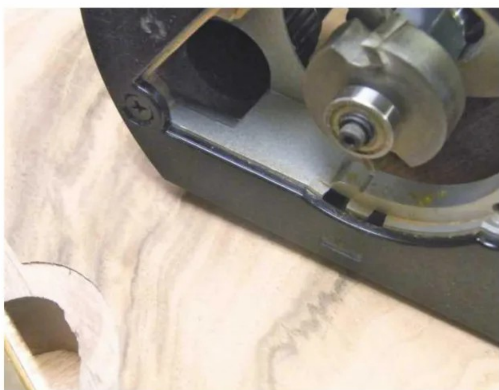
10 Create an 8mm rebate wide round the perimeter, then use a rebate cutter
