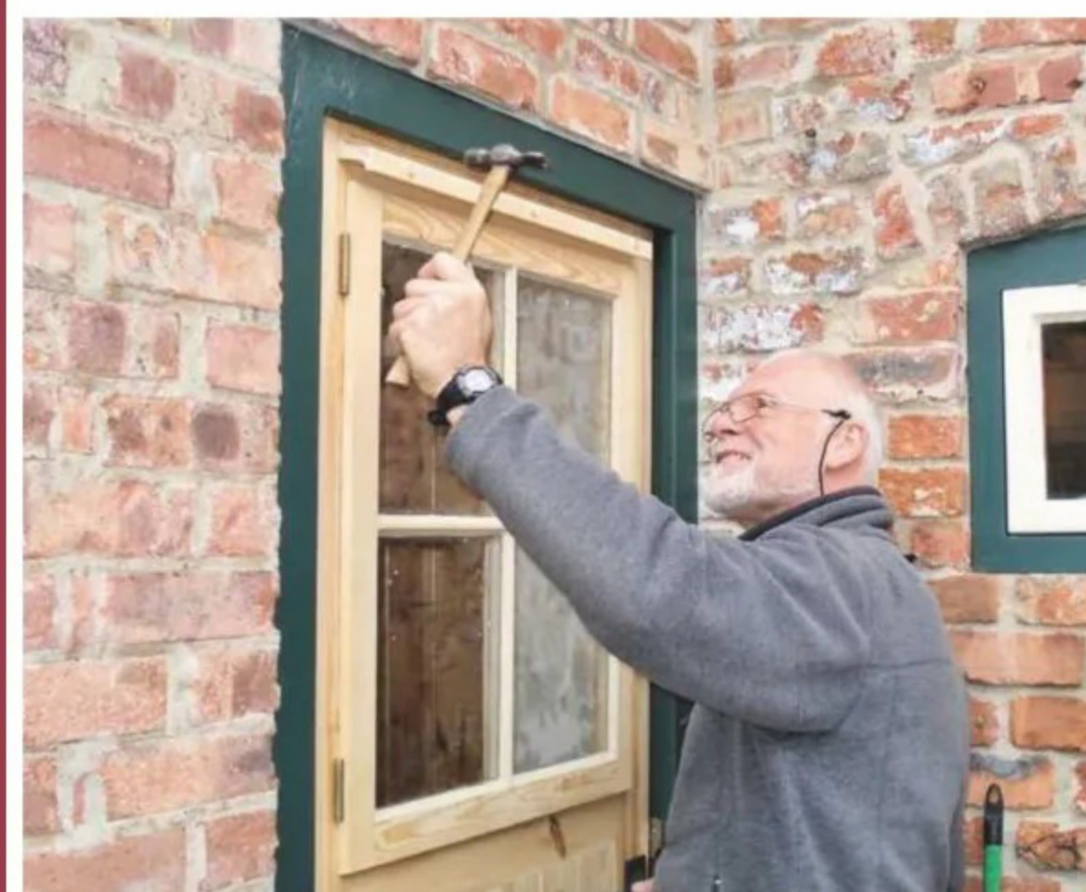
5 ... and the weather moulding with screws that are hidden by pellets
