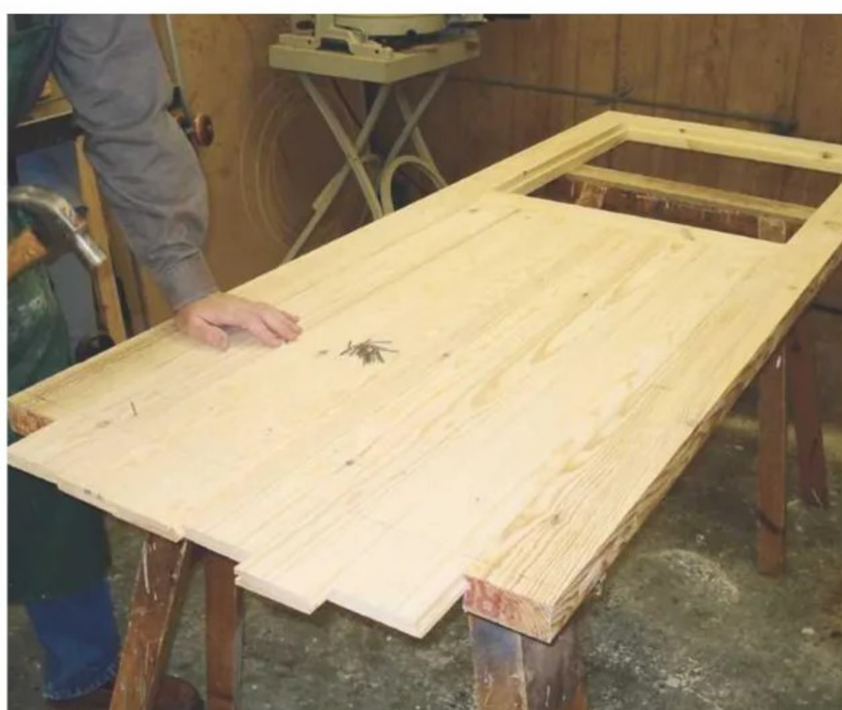
10 Bead-and-butt boarding is secured with 38mm oval nails
