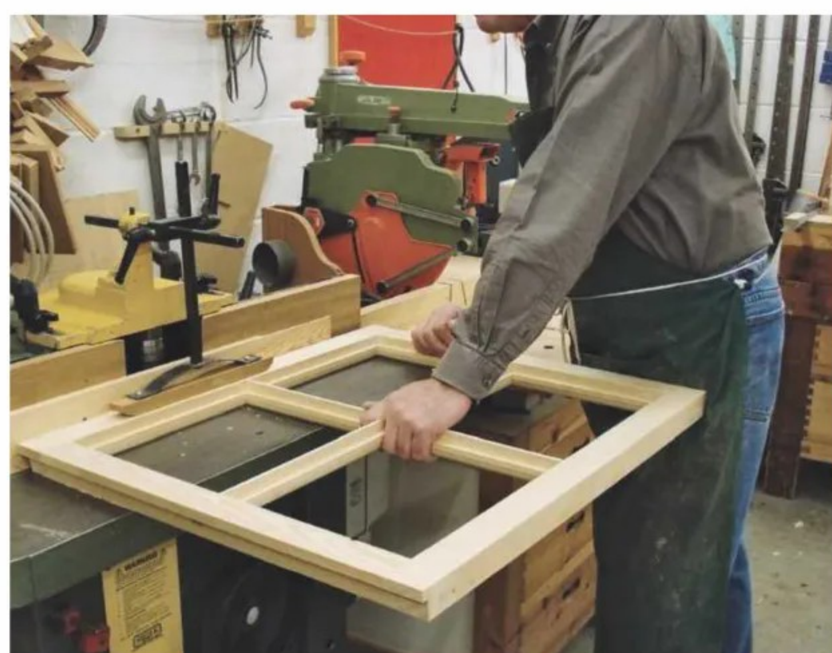
23 The glazing bars are fitted using halving joints, and the outer edges moulded...
