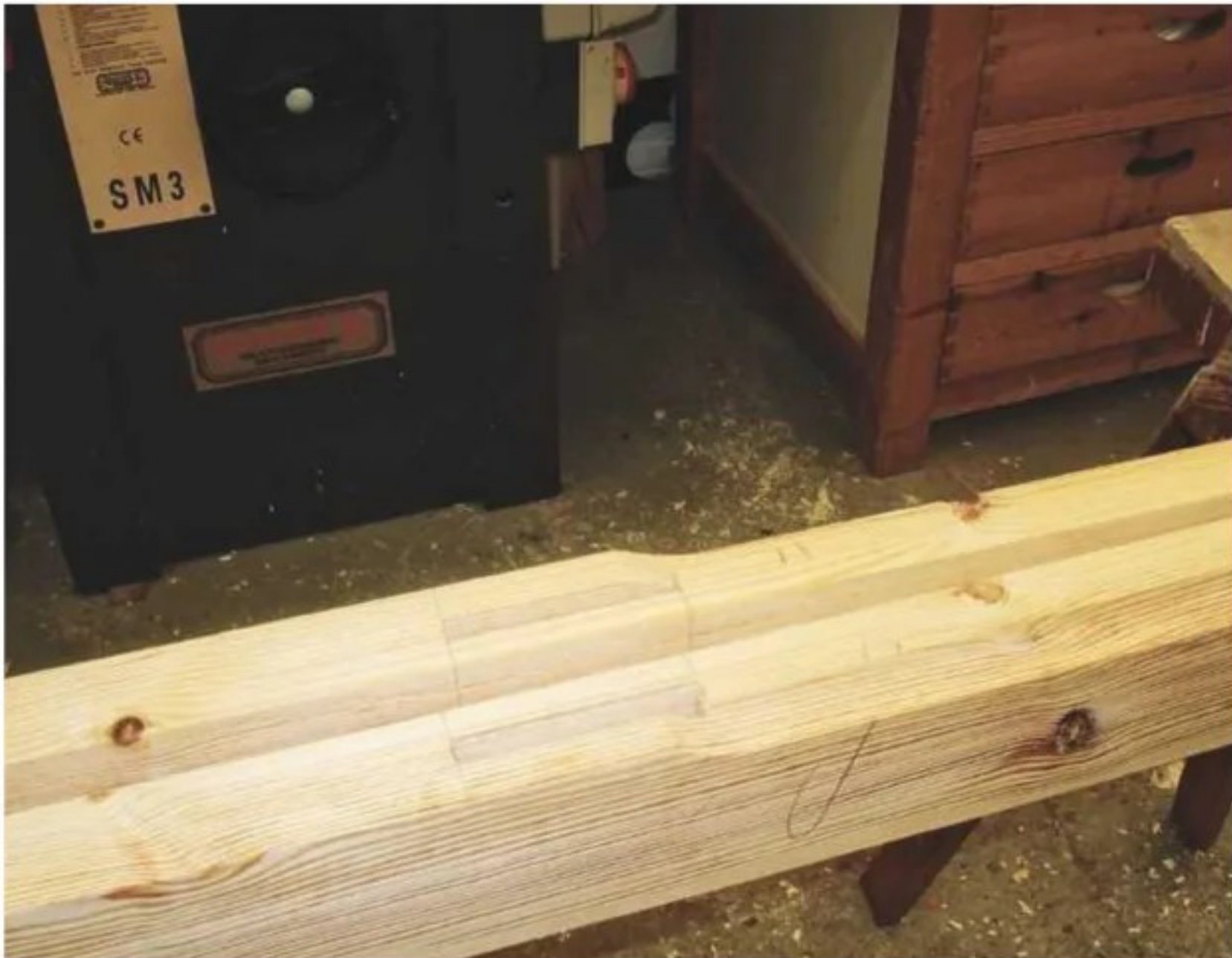
6 At this point, stopped rebates and grooves for the boards were also made
