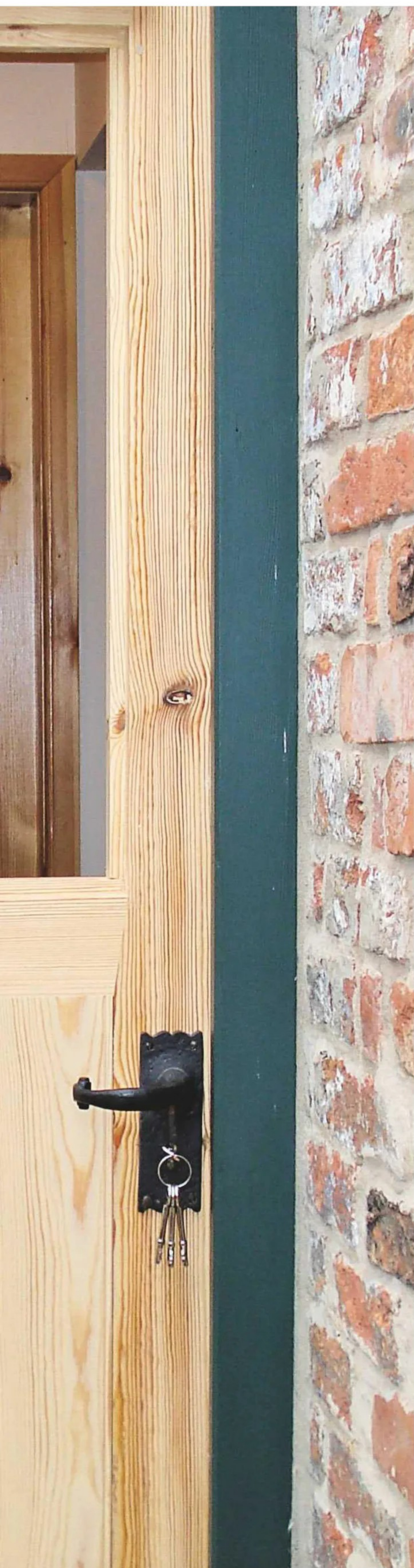
1 I ripped down a 225mm-wide board to make two 100 × 50mm sections for the stiles
