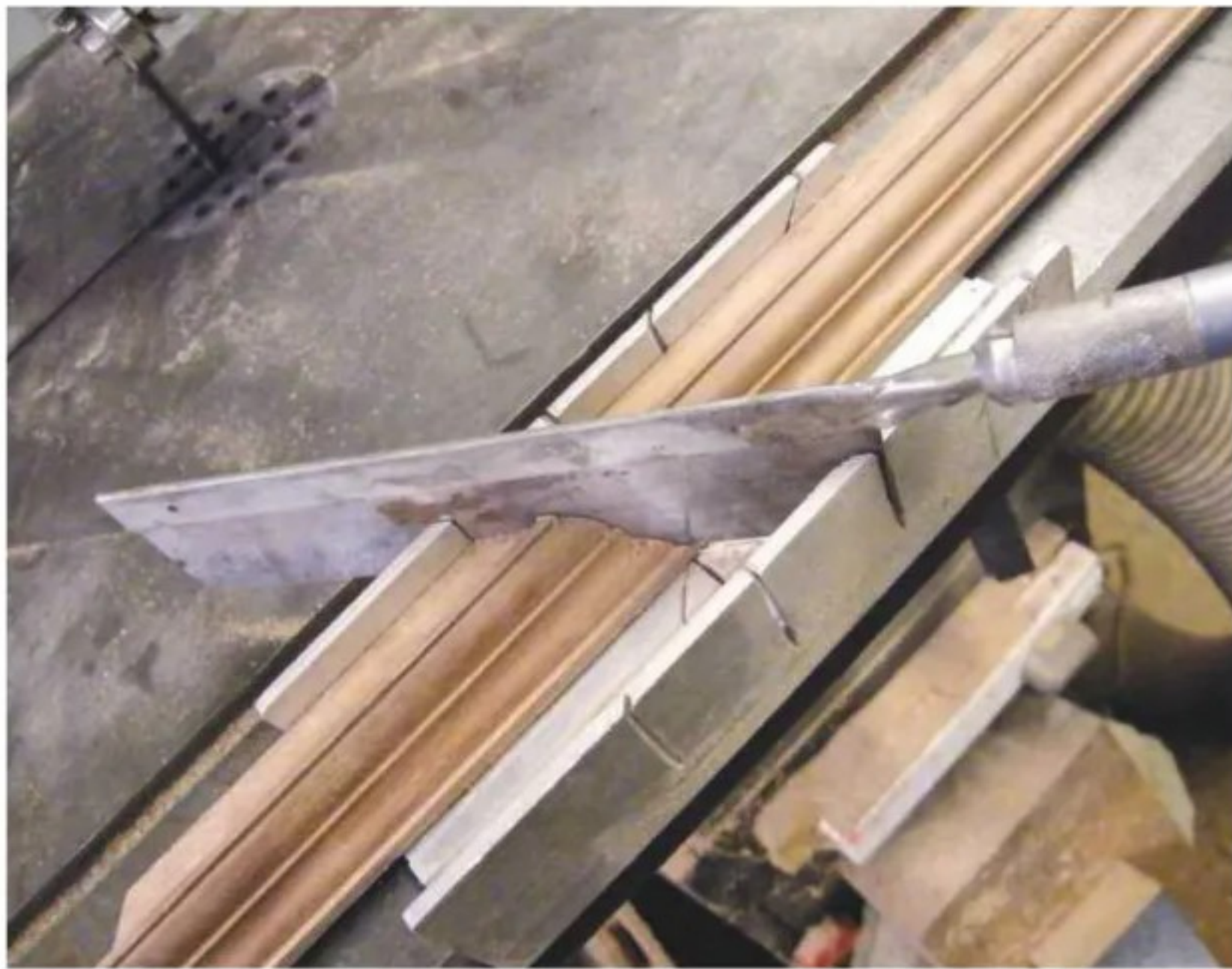
22 Cut the various sections of moulding to length using a small mitre box
