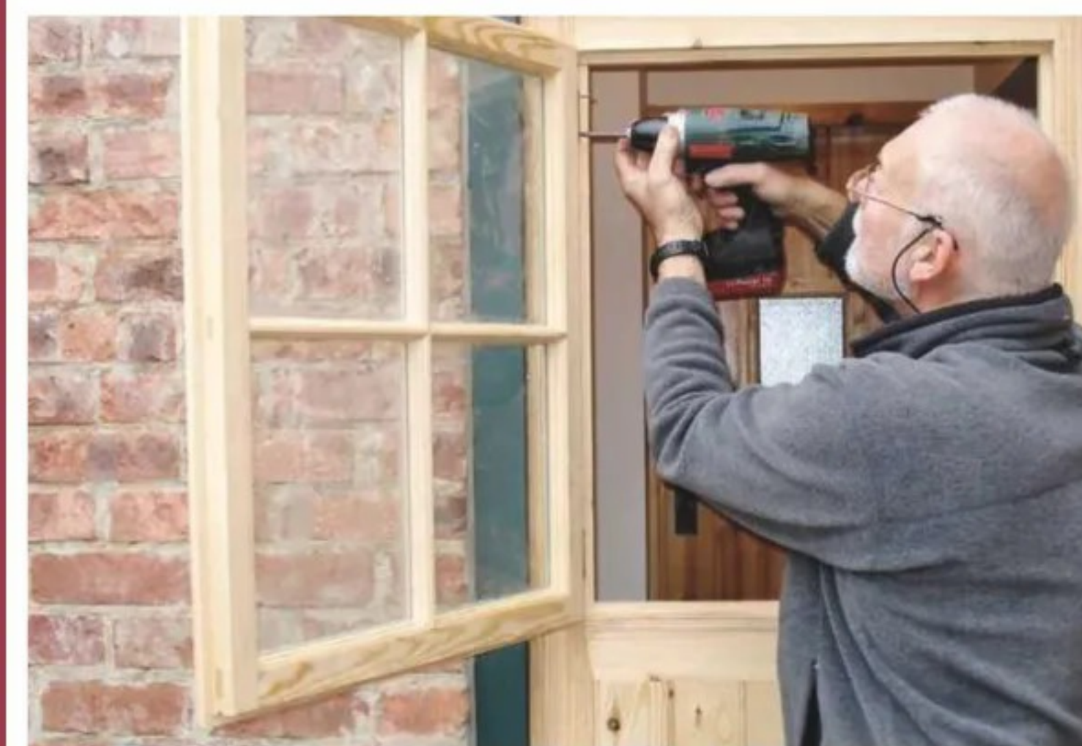
4 Having fitted the glazing, it's time to hang the door...
