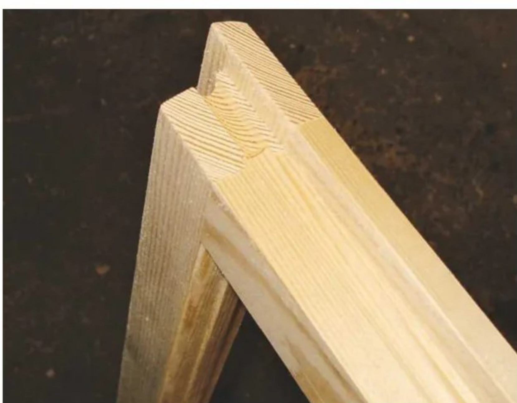
24 ... to create the channel that prevents water ingress
