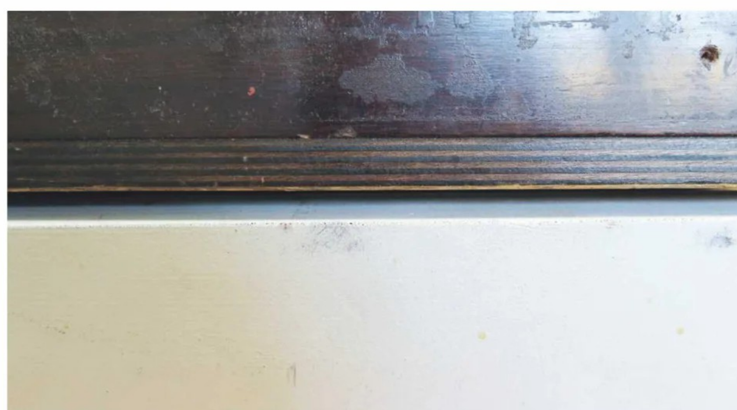
Plywood on the original board was still fit for purpose after some 80+ years
