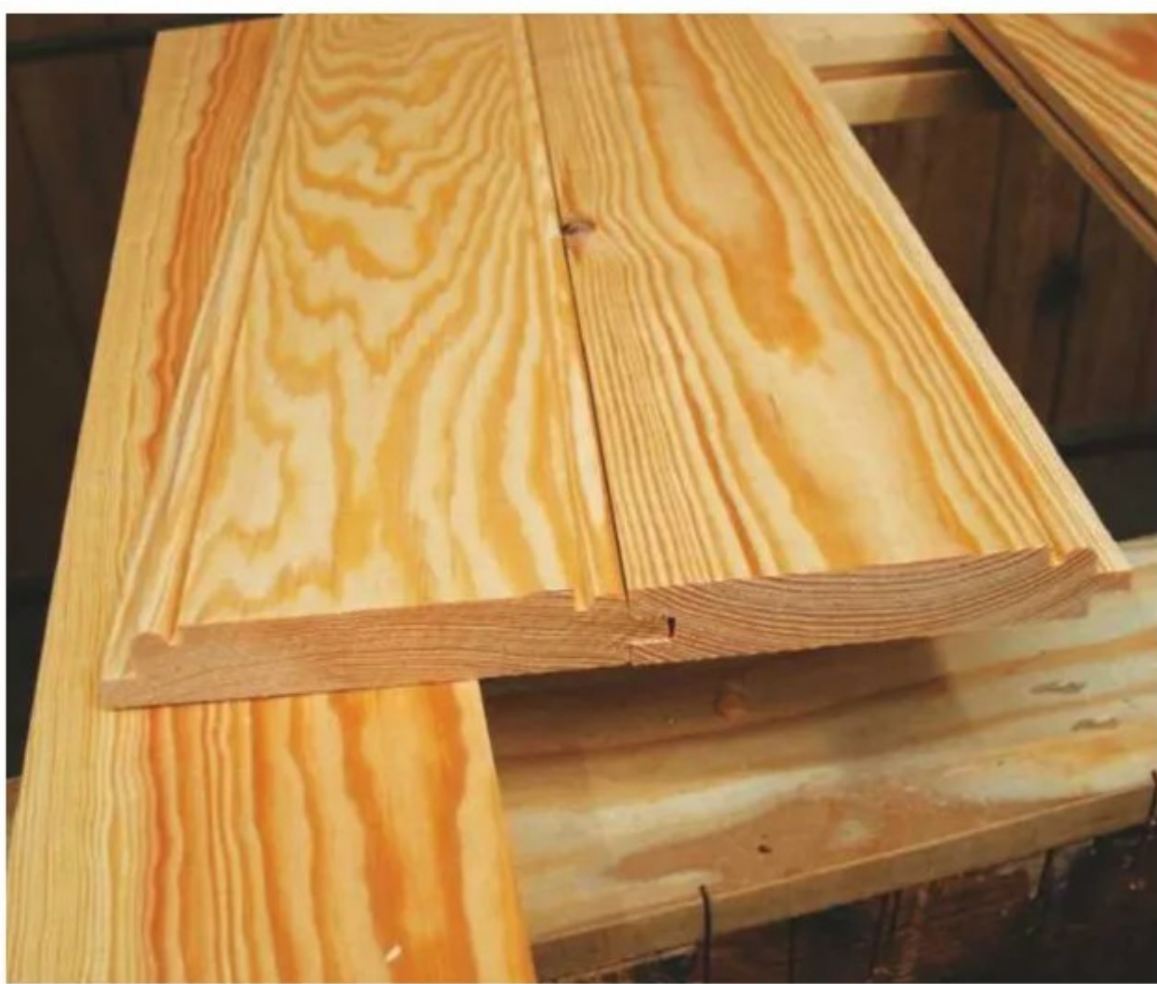
13 The finished butt-and-bead joint – much more sympathetic than TGV
