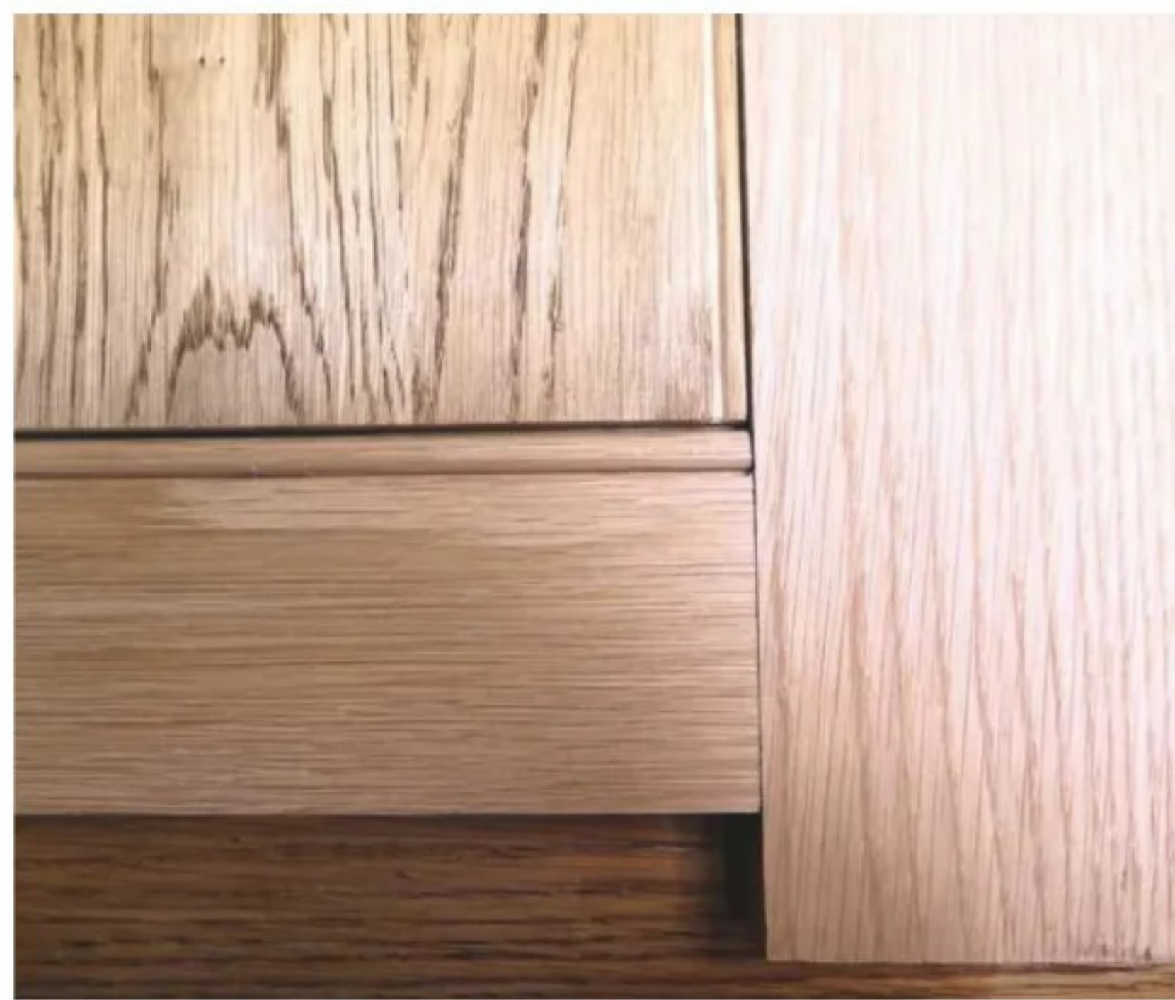
13 Detail showing hand and machine-made corner beads
