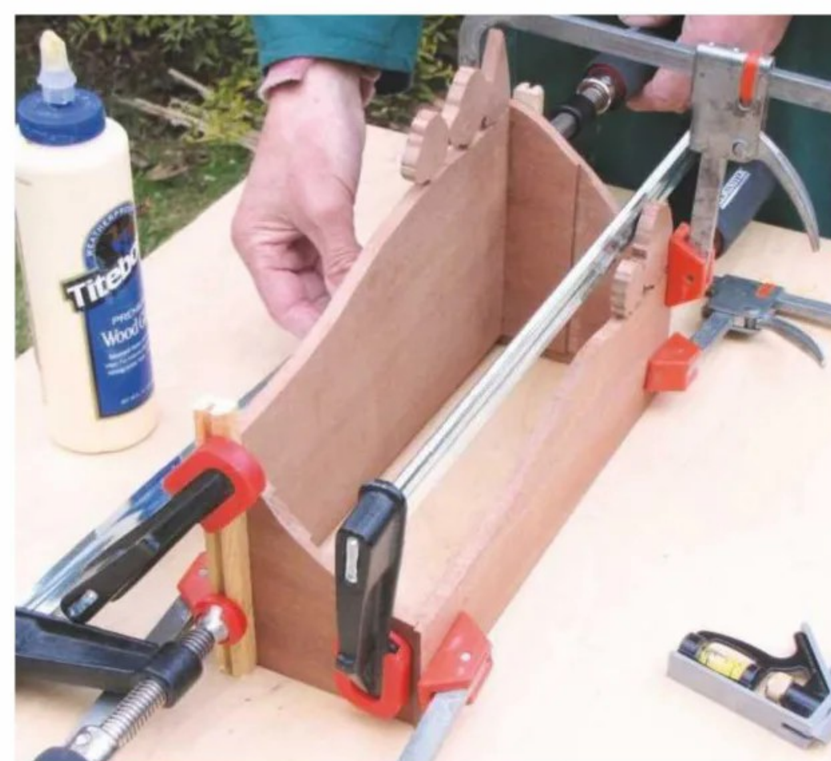
12 Cramp the box together on a flat surface. Check for square, adjusting cramps if necessary
