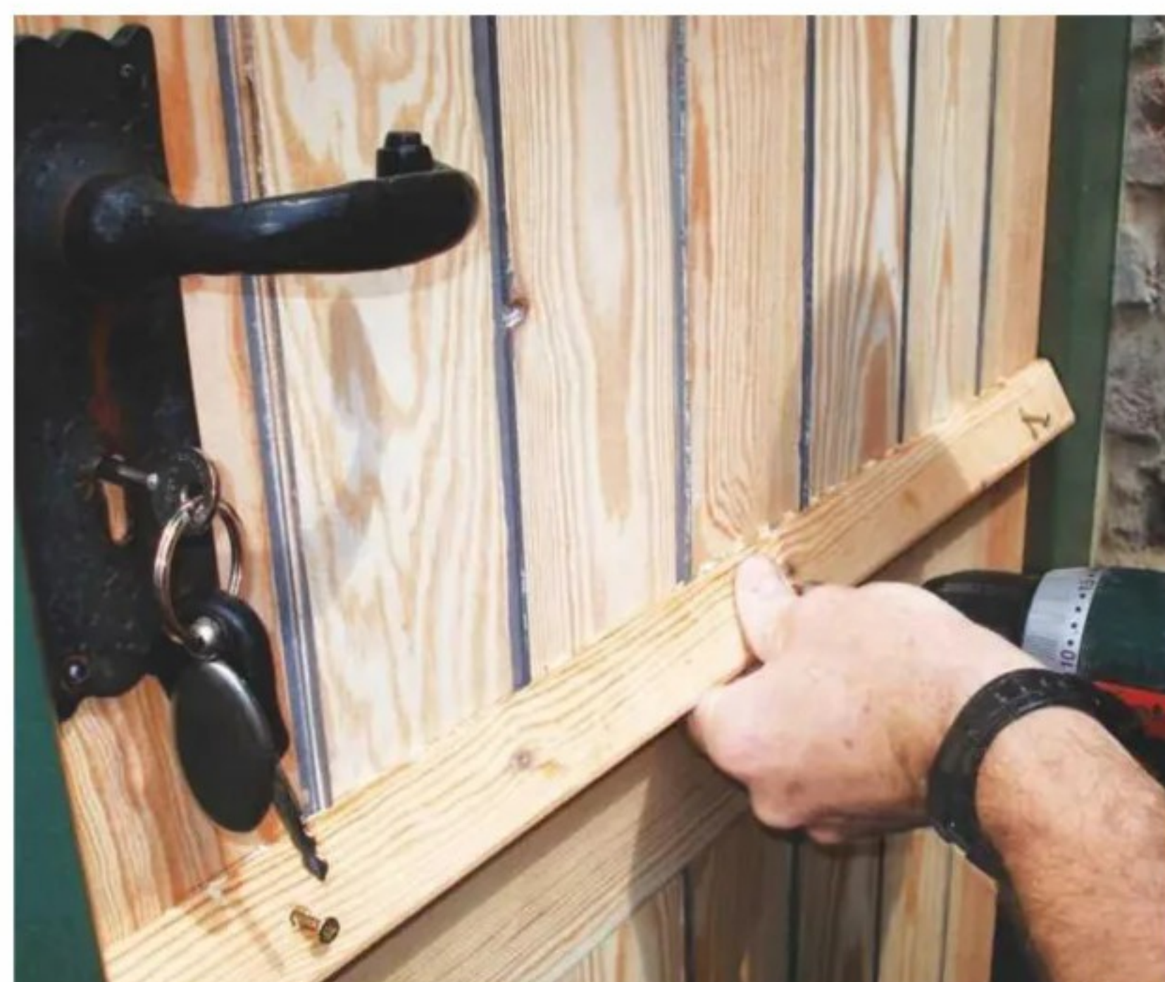
19 Weatherstrips are bedded on putty and screwed in position through the front faces
